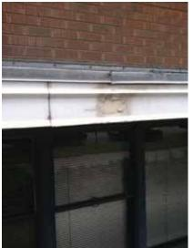
Fig. 2.1.A.51 Flashing with peeling paint at a west window canopy.
