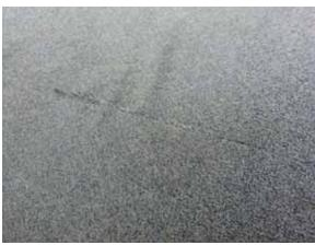
Fig. 3.0.C.16 Typical carpet flooring pulling loose at the seams.
