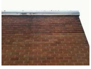
Fig. 2.1.A.11 Deterioration of the mortar and soiling of the brick at the Penthouse walls.
