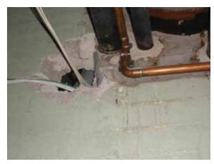
Fig. 2.4.B.3 – Penetrations not fire sealed
