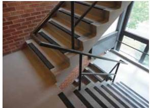
Fig. 2.1.B.5 The spacing between the handrail posts, or guardrails, is not to code, easily allowing passage of a sphere 4 inches in diameter.
