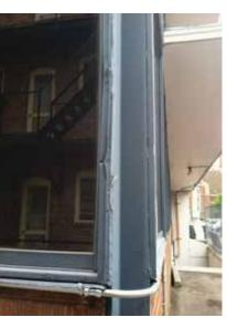
Fig. 2.1.A.24 Damaged window frame with peeling paint.
