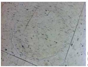
Fig. 3.0.C.12 Damaged linoleum tile noted in the entryway of a Break Room.
