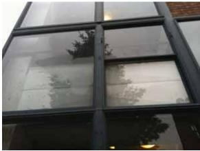
Fig. 2.1.A.29 Fogged glazing at the north side.
