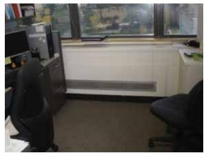
Fig. 2.4.A.18 - Perimeter units blocked by office partitions
