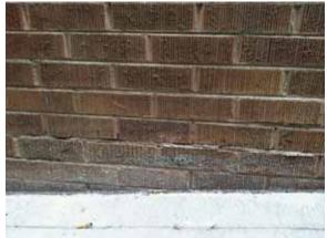
Fig. 2.1.A.10 Deterioration of the mortar at the south side.
