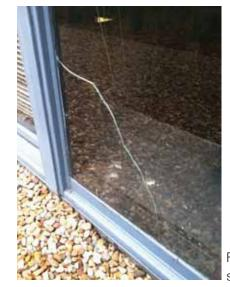
Fig. 2.1.A.26 Broken window at the north side.
