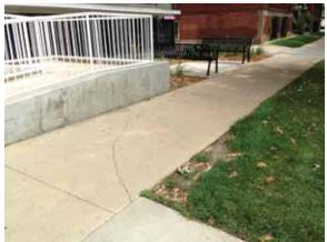
Fig. 2.3.A.7 Sidewalk Crack, Recommended for Replacement
