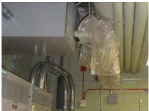
Fig. 2.4.B.2 – Plastic keeping water from electrical gear
