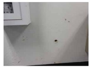
Fig. 3.0.C.9 Water damage at wall near the drinking fountain outside of the Women's Restroom on the Fourth Floor.
