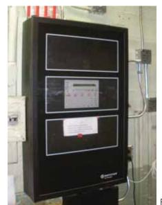
Fig. 2.4.A.4 – Fire alarm control panel
