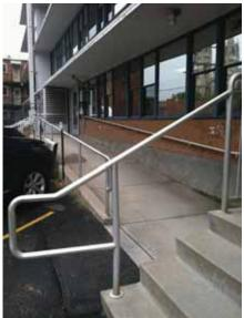
Fig. 2.1.B.7 Water accumulating at the East Entrance ramp.
