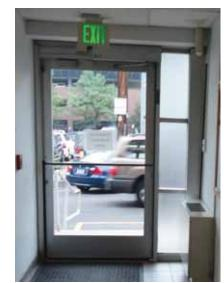
Fig. 2.1.A.31 Exterior door with areas of deteriorated or missing weather stripping at the east side.
