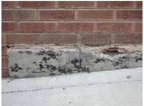
Fig. 2.1.A.13 Deterioration of the mortar and spalling of the concrete foundation at the south side.
