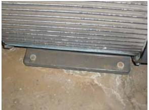
Fig. 2.4.A.12 - Condenser water pump motor installed directly on floor
