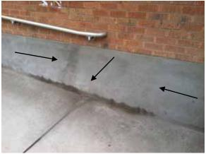
Fig. 2.1.A.18 Cracks in concrete foundation along the ramp at the east entrance where there also appeared to be evidence of standing water.
