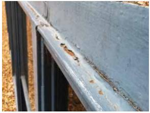
Fig. 2.1.A.23 Corroded window frame with peeling paint.
