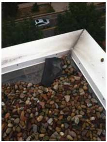
Fig. 2.1.A.36 Spot where the membrane is loose on the roof.
