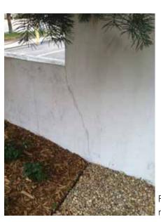
Fig. 2.1.A.56 Crack in the northeast retaining wall.
