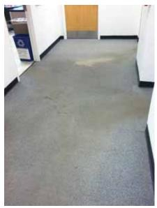
Fig. 3.0.C.15 Typical soiled and stained carpet flooring.
