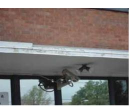
Fig. 2.1.A.52 Flashing with peeling paint at the east entrance canopy.
