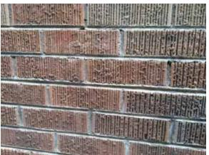
Fig. 2.1.A.8 Minor deterioration of the mortar between the bricks.
