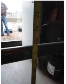
Fig. 2.1.B.3 Measurement to top of railing above finish floor at the Roof Level landing is approximately 31-3/4 inches.
