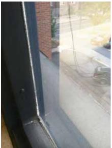
Fig. 2.1.A.22 Single pane window with no thermal break.
