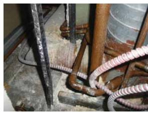
Fig. 2.4.A.19 - Un-insulated piping in the riser
