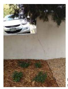
Figure Fig. 2.3.B.1 Crack in Retaining Wall
