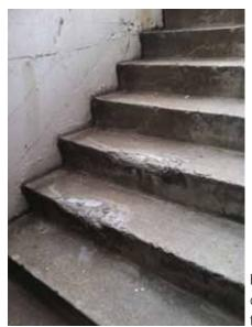
Fig. 2.1.A.54 Damage to exterior concrete stairway on the east side of the building.
