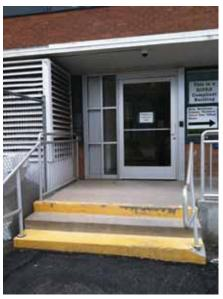
Fig. 2.1.A.55 Spalling of the concrete step outside of the exterior door at the south end of the East Entrance.
