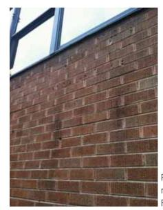
Fig. 2.1.A.1 Holes in the brick at the north side of the building under the First Floor windows.
