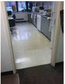
Fig. 3.0.C.11 Discolored linoleum tile in noted in a Break Room.
