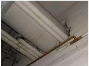
Fig. 2.4.B.4 - Penetrations not fire sealed
