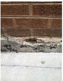
Fig. 2.1.A.14 Deterioration of the mortar and spalling of the concrete foundation at the south side.
