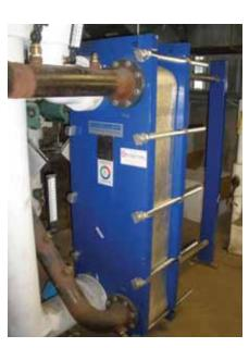
Fig. 2.4.A.15 - Missing insulation on Heat Exchanger Piping
