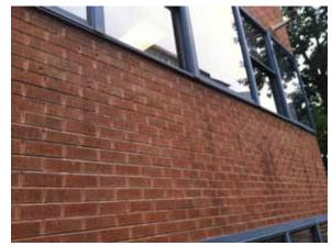
Fig. 2.1.A.2 Holes in the brick at the north side of the building under the First Floor windows.
