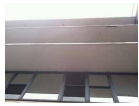
Fig. 2.1.A.50 Canopies over windows on the east side of the building with peeling paint, cracking, and spalling.
