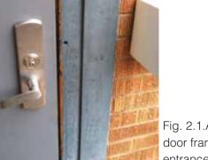
Fig. 2.1.A.33 Soiled and damaged door frame at the north end of the east entrance.
