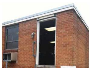
Fig. 2.1.A.20 Peeling paint at the concrete around the perimeter of the Penthouse.
