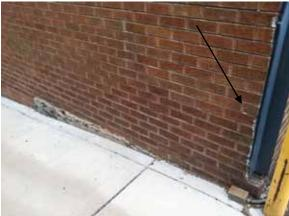
Fig. 2.1.A.5 Minor spalling at the south side of the building, on the east end.
