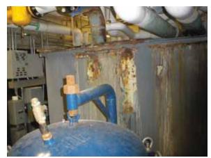
Fig. 2.4.A.10 - Rusting on outside of tower sump
