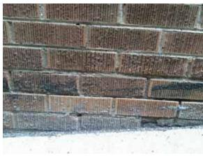
Fig. 2.1.A.9 Deterioration of the mortar at the south side.
