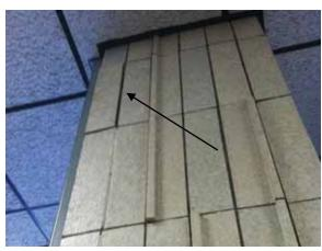
Fig. 3.0.C.6 Masonry veneer pulling away from the walls of the Grant Street Entrance lobby.
