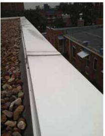
Fig. 2.1.A.42 Warping parapet coping.
