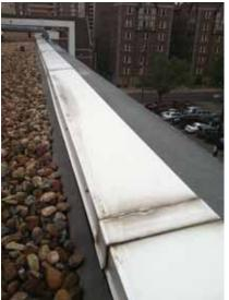
Fig. 2.1.A.41 Typical parapet coping with deteriorating sealant along the joints and with evidence of standing water.
