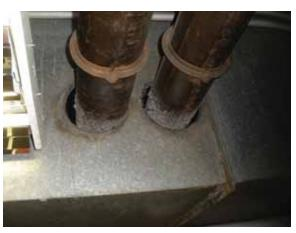
Fig. 2.4.A.21 – Pipe penetration through ductwork/no sealing around pipes
