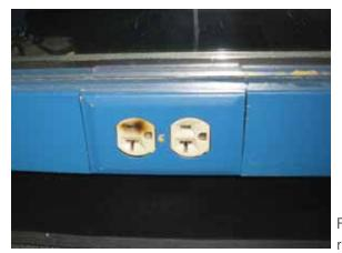
Fig. 2.4.A.5 – Burned out receptacle
