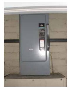
Fig. 2.4.B.1 – Disconnect switch without proper working space
