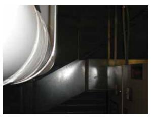
Fig. 2.4.B.6 – Ductwork in front of chiller control panel
