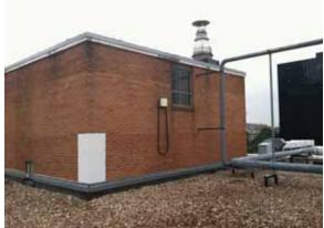
Fig. 2.1.A.12 Deterioration of the mortar and soiling of the brick at the Penthouse walls.
