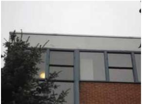
Fig. 2.1.A.19 Peeling paint at the concrete cap around the perimeter of the roof.
