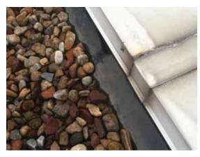
Fig. 2.1.A.40 Typical deteriorating sealant found along the joints of the parapet coping.
