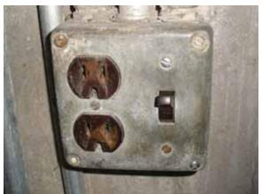
Fig. 2.4.A.6 – Receptacle and switch past useful life
