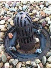
Fig. 2.1.A.37 Drain cover showing signs of corrosion.
