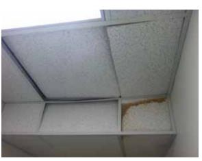
Fig. 3.0.C.3 Damaged 2x4 acoustic ceiling tiles.
