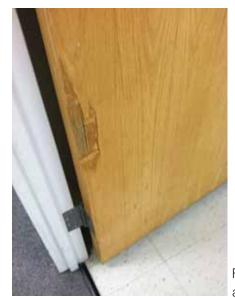
Fig. 3.0.C.19 Damaged door noted at a Break Room.
