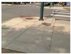
Fig. 2.3.A.8 Broken Site Concrete, Recommended for Replacement
