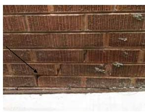
Fig. 2.1.A.4 Cracking along the joints between the brick at the south side.
