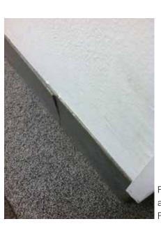
Fig. 3.0.C.18 Vinyl baseboard pulling away from the wall on the Basement Floor.
