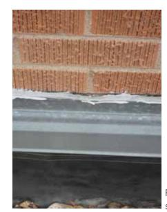
Fig. 2.1.A.39 Typical deteriorating sealant found along the flashing.
