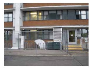
Fig. 2.4.A.22 – Outside air intake at ground level
