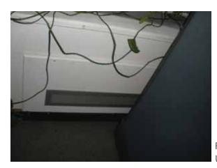
Fig. 2.4.A.17 – Induction Unit blocked
