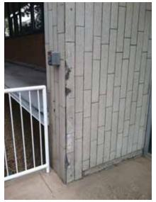
Fig. 2.1.A.21 Damaged and missing masonry veneer at the Grant Street Entrance.
