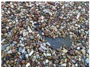
Fig. 2.1.A.34 Area of thin ballast leaving the roof membrane exposed on the roof.
