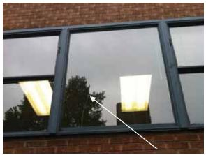
Fig. 2.1.A.27 Broken window at the north side.
