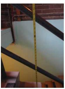
Fig. 2.1.B.4 Measurement to top of railing above the stair nosing is approximately 29-1/2 inches.
