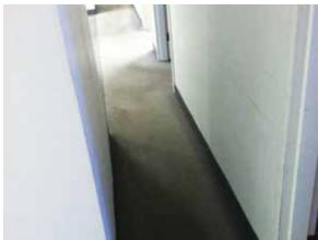
Fig. 3.0.C.7 Areas of scuffed paint on the painted gypsum board walls.
