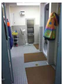
Fig. 2.1.C.3 Mats on the floor outside of the showers provide issues with approaching the accessible toilet compartment.
