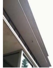
Fig. 2.1.A.48 Canopies over windows on the west side of the building with peeling paint, cracking, and spalling.
