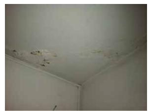
Fig. 3.0.C.4 Water damage to the ceiling along the west side of Room 026
