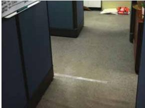
Fig. 3.0.C.17 Typical carpet flooring in generally poor condition and with tape covering the loose seams.
