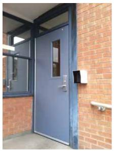
Fig. 2.1.A.32 Soiled and damaged door frame at the north end of the east entrance.
