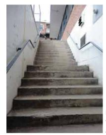
Fig. 2.1.A.53 Exterior concrete stairway on the east side of the building with cracking and spalling.
