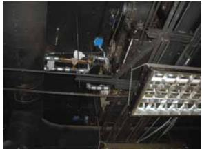
Fig. 2.4.A.20 - No belt guard provided for AHU
