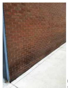
Fig. 2.1.A.7 Soiled brick at the south side of the building at grade level.
