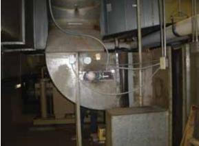
Fig. 2.4.A.14 - SA duct from AHU
