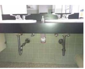
Fig. 2.1.C.2 Accessible lavatory pipes without protective insulation.
