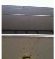
Fig. 2.1.A.46 Water damage observed underneath the Grant Street Entrance canopy.
