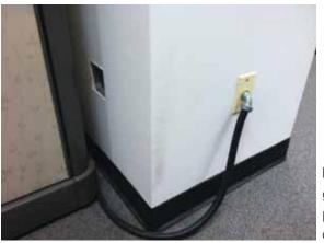
Fig. 3.0.C.8 Unpatched gypsum board at a previously removed wall outlet on the Third Floor.
