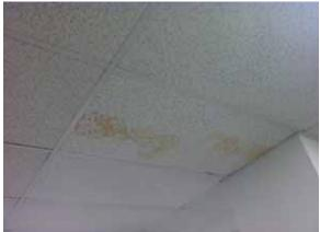
Fig. 3.0.C.2 Stained 2x4 acoustic ceiling tiles.
