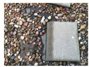
Fig. 2.1.A.35 Area of thin ballast leaving the roof membrane exposed on the roof.
