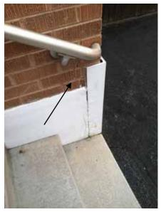
Fig. 2.1.A.3 Cracking along brick joints at the north side of the east building entrance.
