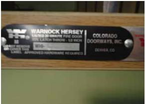
Fig. 2.1.B.1 Fire rating label on interior exit stairway door.
