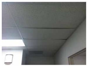
Fig. 3.0.C.1 Sagging 2x4 acoustic ceiling tiles.
