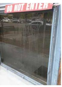
Fig. 2.1.A.30 Bent window frame at the southwest corner with corrosion at the base.
