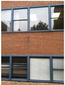
Fig. 2.1.A.6 Typical instance of soiled brick found under the windows.
