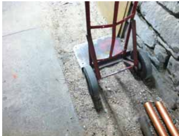
Fig. 3.1.C.49 Missing concrete pavers observed in a few locations throughout the Sub-basement Floor.
