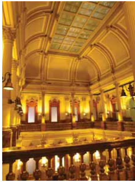
Zone 2 Original Interior Circulation: Interior skylight at the top of the east atrium
