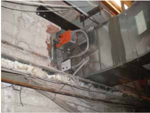
Fig. 2.4.A.42 – Opening in wall
