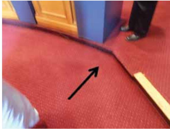
Fig. 2.4.A.27 – Supply air grille
