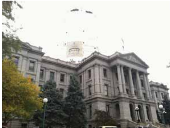
Front/West Elevation of the State Capitol
