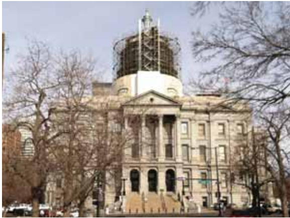
South Elevation of the State Capitol
