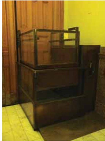
Fig. 2.1.C.8 Wheelchair lift observed on the Second Floor outside of the Senate Gallery.
