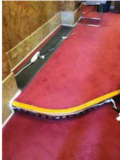
Fig. 3.1.C.42 Electrical cords running loosely across the floor of the Old Supreme Court Chambers and creating a potential tripping hazard.
