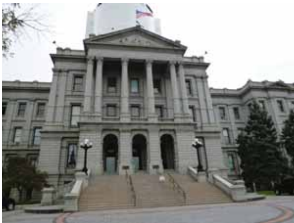
Zone 1 Exterior Facade: West elevation
