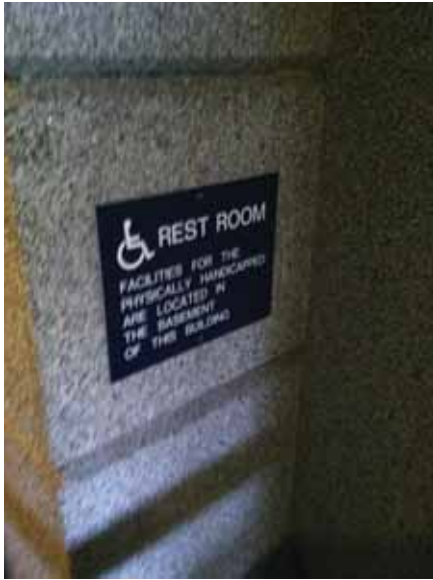
Fig. 2.1.C.1 Accessible public restroom facilities are located on the Basement Floor.
