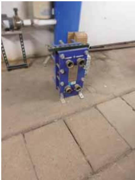
Fig. 2.4.A.37 – Steam condensate heat recharger
