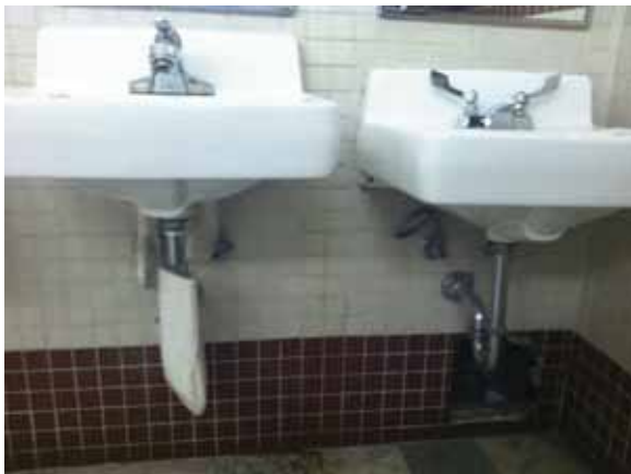
Fig. 3.1.C.20 Damage to the wall observed in the Women's Accessible Restroom on the Basement Floor.
