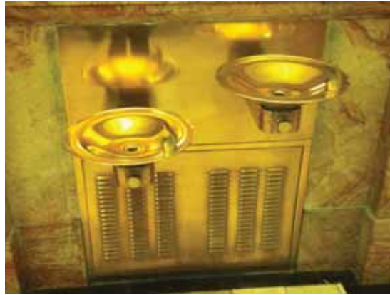
Fig. 2.1.C.3 Typical accessible drinking fountain observed during the site survey visit.
