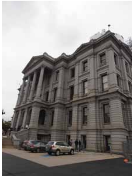
Fig. 2.4.A.39 – Window AC units
