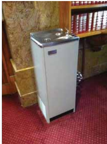
Fig. 2.1.C.4 Non-accessible drinking fountain noted in the Senate Gallery.
