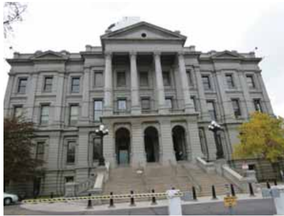
Zone 1 Exterior Facade: North elevation
