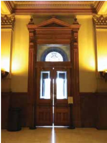
Fig. 2.1.A.21 Interior doors at the entrance vestibules were generally noted to have air gaps between the door slabs.
