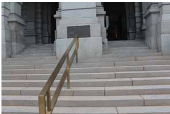
Figure 2.3.A.2 – East Entrance Stairs
