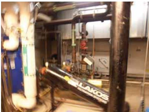
Fig. 2.4.A.38 – Cooling tower and heat recharger
