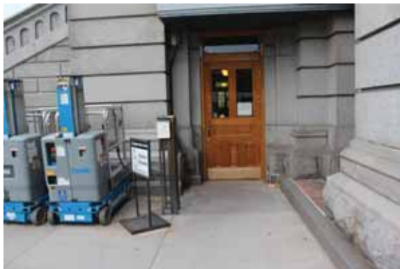
Figure 2.3.A.3 – South Accessible Entrance
