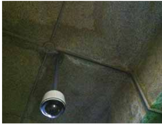
Fig. 3.1.C.3 Water damage noted at the granite cladding on the ceiling of the south accessible entrance vestibule on the Basement Floor.
