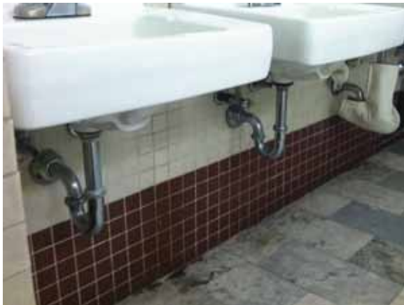
Fig. 3.1.C.19 Generally soiled wall tile noted in the public accessible restrooms on the Basement Floor.
