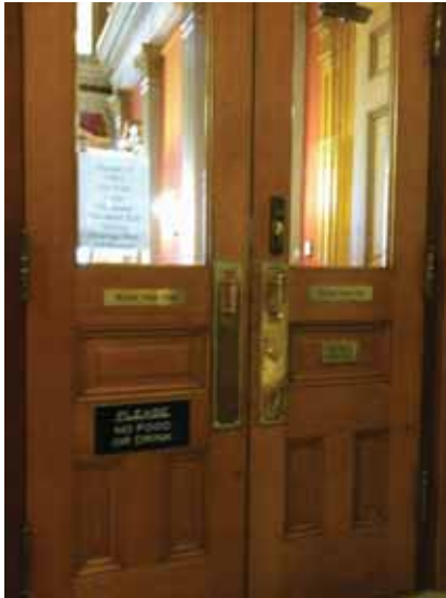
Fig. 2.1.C.10 Inconsistent signage styles observed throughout.
