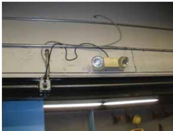
Fig. 2.4.A.10 – Twin-head wall pack emergency luminaire
