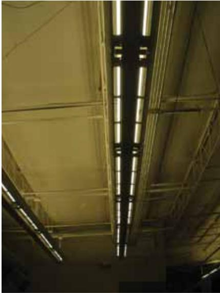
Fig. 2.4.A.5 – Linear luminaires located in the open office space
