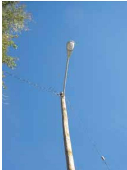
Fig. 2.4.A.9 – Pole mounted metal halide luminaire
