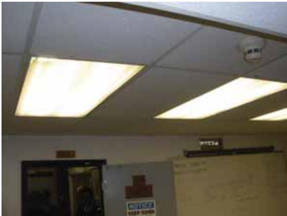
Fig. 2.4.A.6 – Recessed lensed luminaires located in the student class room
