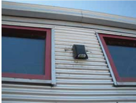
Fig. 2.4.A.8 – Wall mounted LED luminaire
