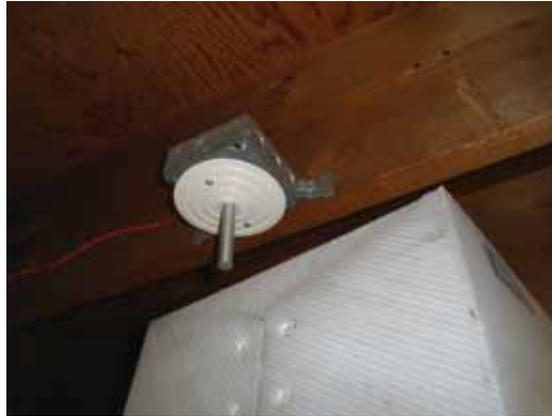
Fig. 2.4.A.14 – Heat detector
