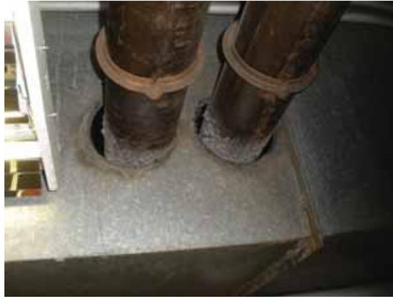
Fig. 2.4.A.21 – Pipe penetration through ductwork/no sealing around pipes
