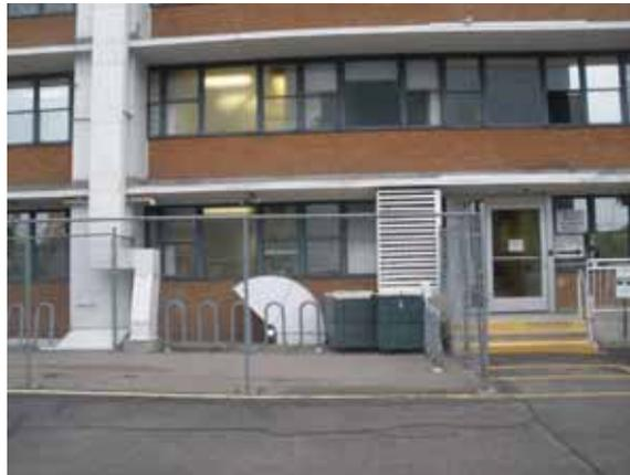
Fig. 2.4.A.22 – Outside air intake at ground level
