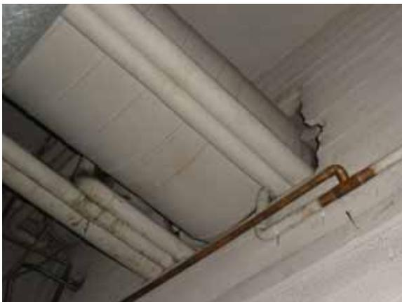
Fig. 2.4.B.4 - Penetrations not fire sealed
