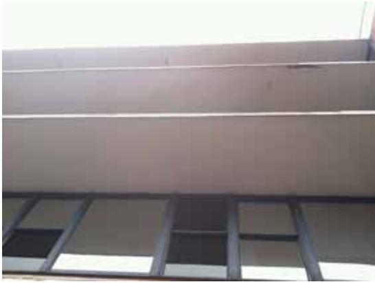
Fig. 2.1.A.50 Canopies over windows on the east side of the building with peeling paint, cracking, and spalling.
