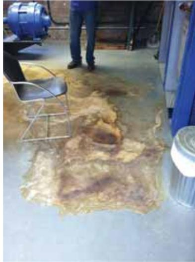
Fig. 2.1.A.43 Signs of water damage on the floor of the Penthouse.
