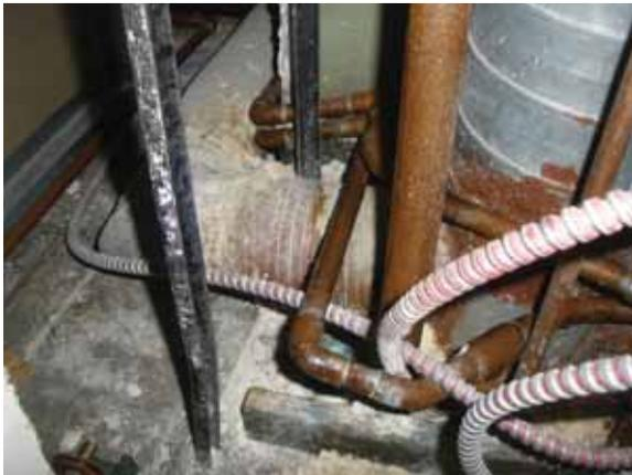
Fig. 2.4.A.19 - Un-insulated piping in the riser
