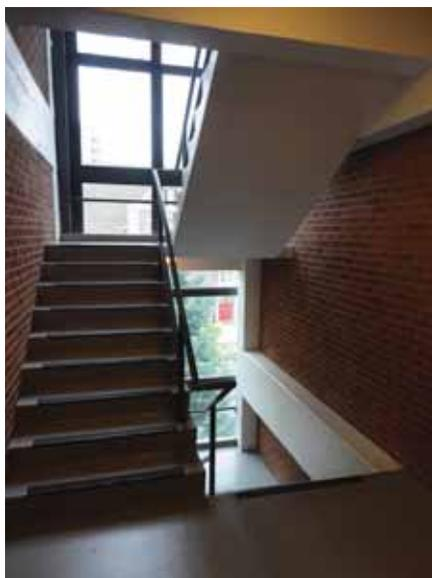
Fig. 2.1.B.2 Handrails currently exist on only one side of the stairs.
