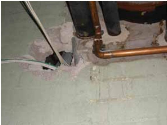
Fig. 2.4.B.3 – Penetrations not fire sealed
