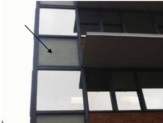
Fig. 2.1.A.16 Cracked concrete panel at the southeast corner.
