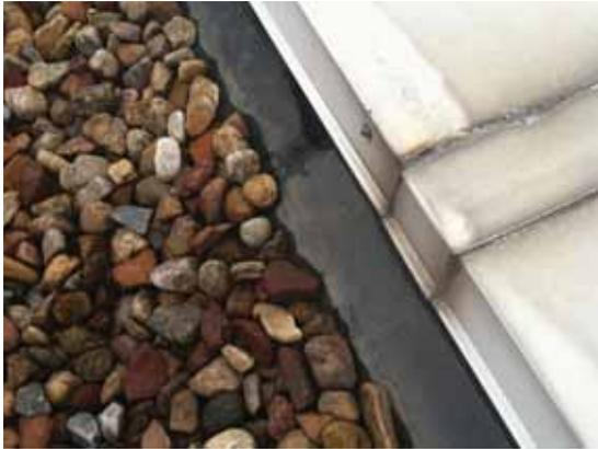
Fig. 2.1.A.40 Typical deteriorating sealant found along the joints of the parapet coping.
