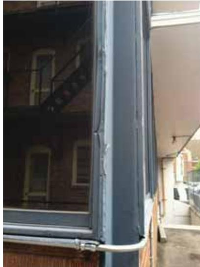
Fig. 2.1.A.24 Damaged window frame with peeling paint.
