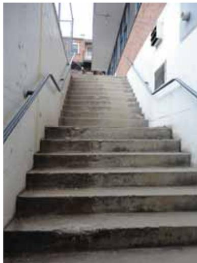
Fig. 2.1.A.53 Exterior concrete stairway on the east side of the building with cracking and spalling.
