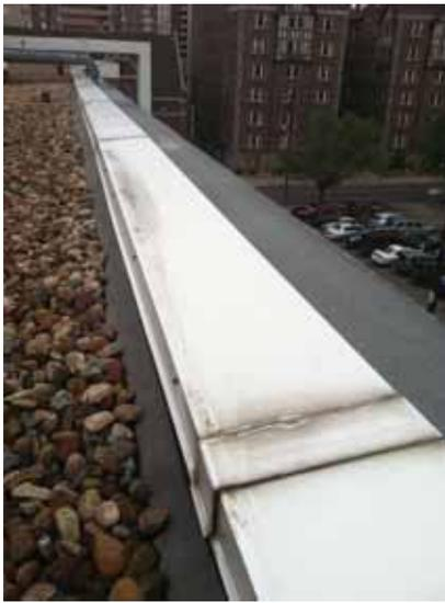
Fig. 2.1.A.41 Typical parapet coping with deteriorating sealant along the joints and with evidence of standing water.
