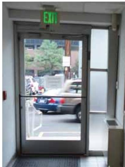
Fig. 2.1.A.31 Exterior door with areas of deteriorated or missing weather stripping at the east side.
