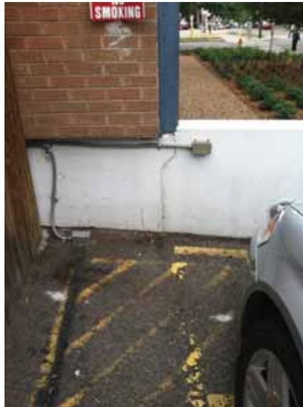
Fig. 2.1.A.57 Crack in the northeast retaining wall.
