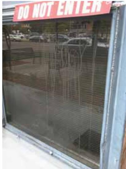
Fig. 2.1.A.30 Bent window frame at the southwest corner with corrosion at the base.
