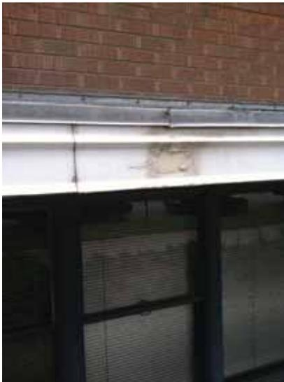
Fig. 2.1.A.51 Flashing with peeling paint at a west window canopy.
