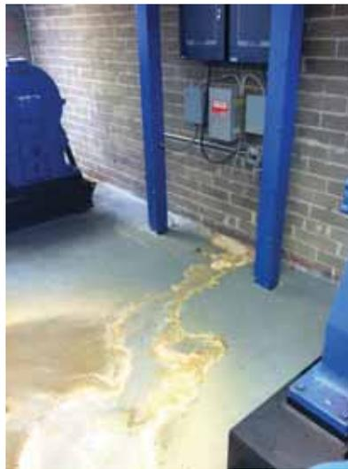
Fig. 2.1.A.44 Signs of water damage on the floor of the Penthouse.
