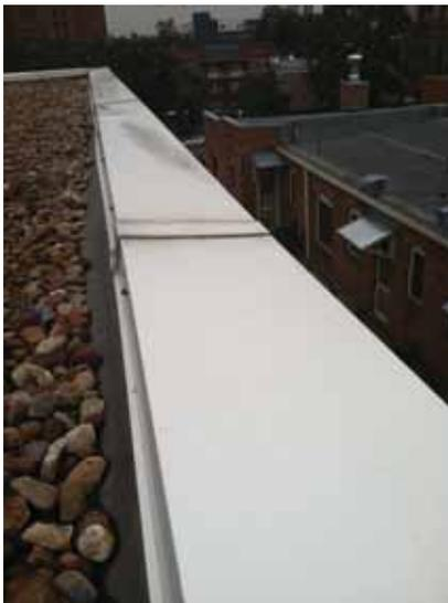
Fig. 2.1.A.42 Warping parapet coping.
