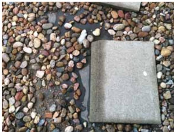
Fig. 2.1.A.35 Area of thin ballast leaving the roof membrane exposed on the roof.
