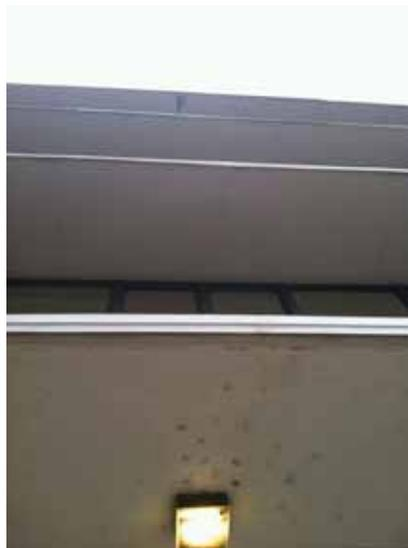
Fig. 2.1.A.46 Water damage observed underneath the Grant Street Entrance canopy.
