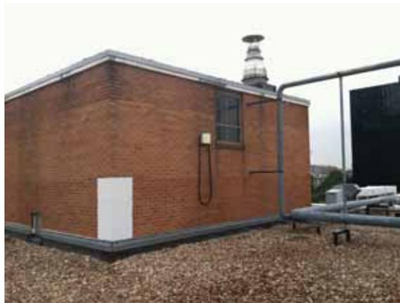
Fig. 2.1.A.12 Deterioration of the mortar and soiling of the brick at the Penthouse walls.
