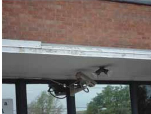
Fig. 2.1.A.52 Flashing with peeling paint at the east entrance canopy.
