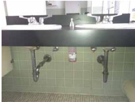
Fig. 2.1.C.2 Accessible lavatory pipes without protective insulation.
