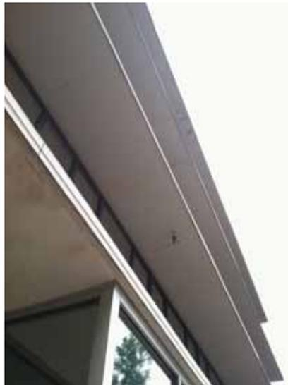
Fig. 2.1.A.48 Canopies over windows on the west side of the building with peeling paint, cracking, and spalling.
