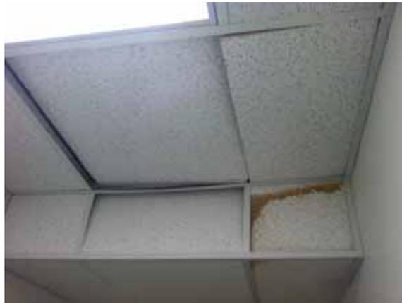
Fig. 3.0.C.3 Damaged 2x4 acoustic ceiling tiles.
