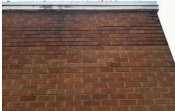
Fig. 2.1.A.11 Deterioration of the mortar and soiling of the brick at the Penthouse walls.
