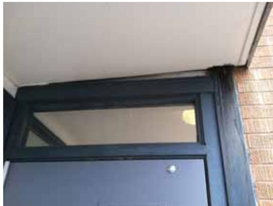
Fig. 2.1.A.47 Canopy leaking at the north end of the East Entrance.
