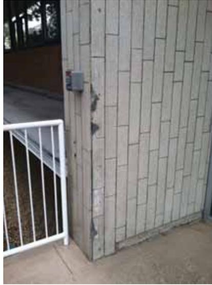
Fig. 2.1.A.21 Damaged and missing masonry veneer at the Grant Street Entrance.
