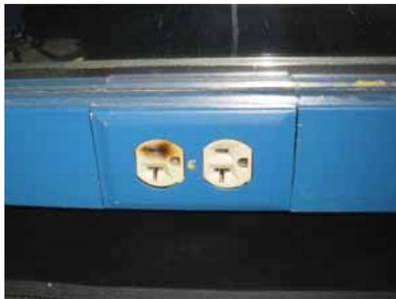
Fig. 2.4.A.5 – Burned out receptacle
