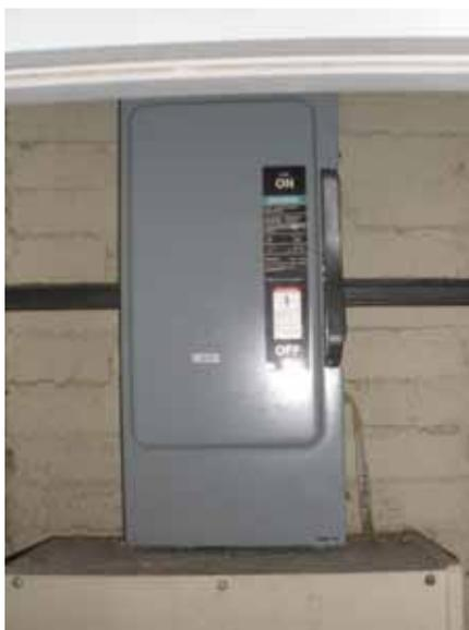
Fig. 2.4.B.1 – Disconnect switch without proper working space
