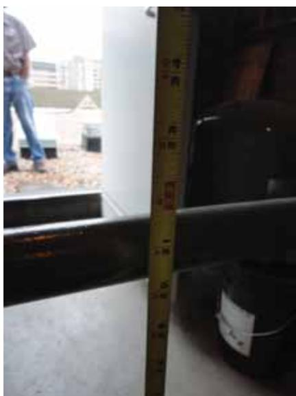
Fig. 2.1.B.3 Measurement to top of railing above finish floor at the Roof Level landing is approximately 31-3/4 inches.
