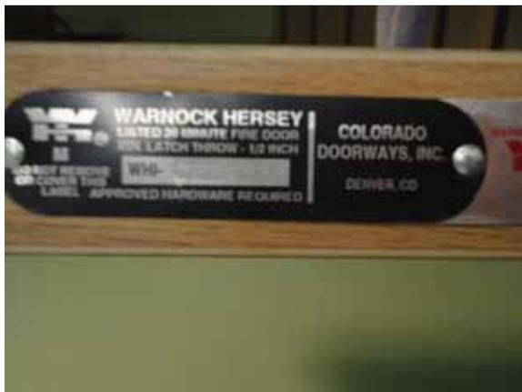
Fig. 2.1.B.1 Fire rating label on interior exit stairway door.
