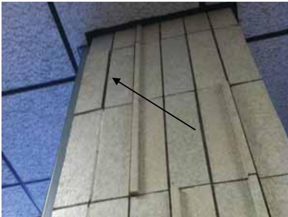
Fig. 3.0.C.6 Masonry veneer pulling away from the walls of the Grant Street Entrance lobby.
