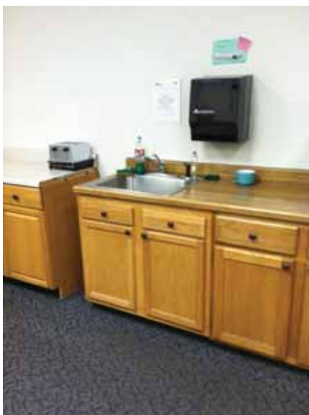
Fig. 2.1.C.2 Non-accessible sink observed in the Break Room on the south side of the building.
