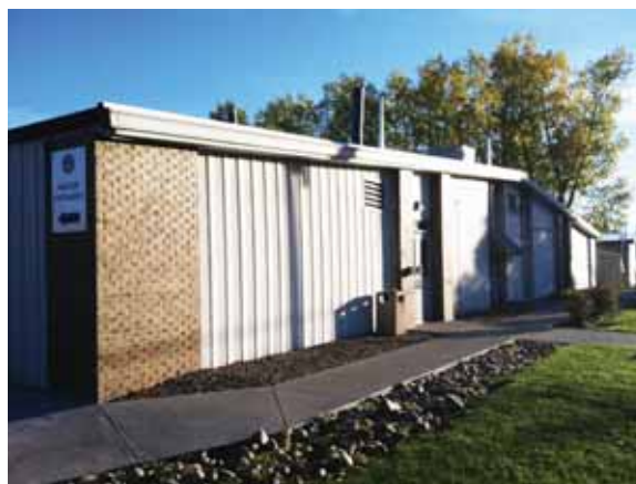
Front/South Elevation of the North Campus West Building
