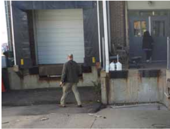
Fig. 2.1.A.50 Corrosion observed at the northwest loading dock.
