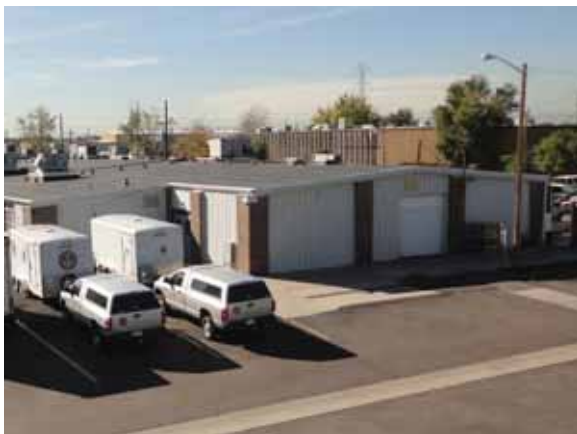
Back/North Elevation of the North Campus West Building
