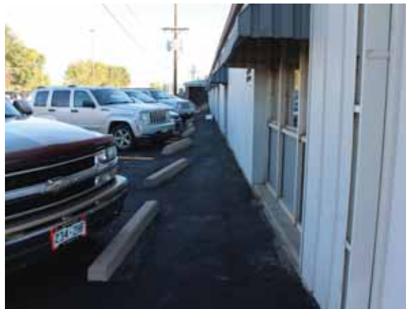
Figure 2.3.B.1 – Building Perimeter, Slopes Away
