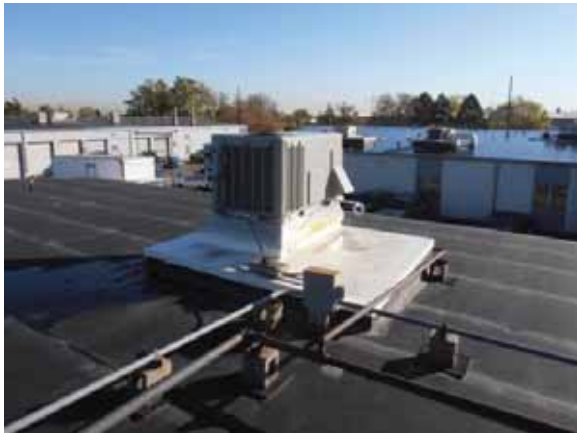
Fig. 2.4.A.18 – New Trane unit installation
