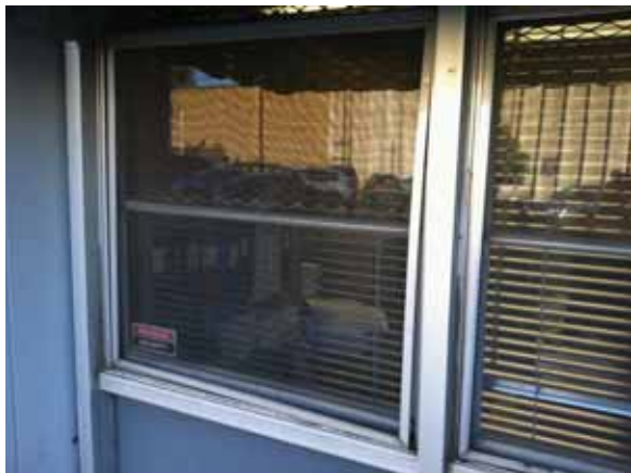
Fig. 2.1.B.12 Honeywell Security sign observed on a few windows around the exterior of the building.
