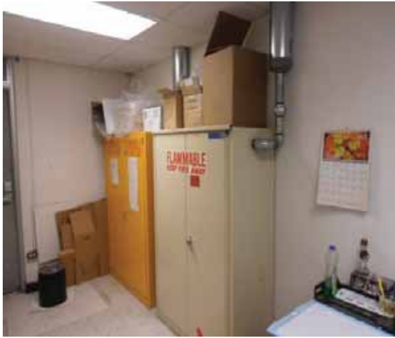
Fig. 2.4.A.23 – Chemical storage area
