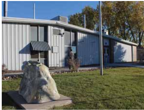
Figure 2.3.A.2 – West Building, South Entrance
