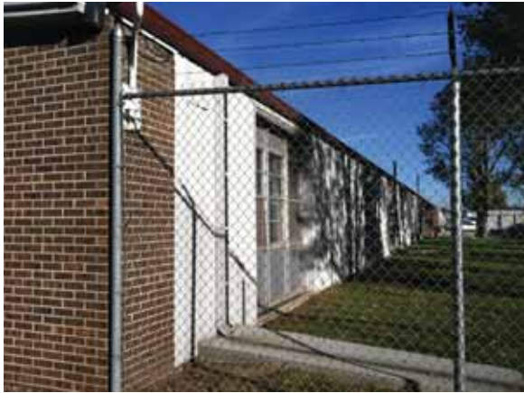
Fig. 2.1.B.11 South fence between the North Campus West Building and the North Campus East Building with barbed wire along the top.
