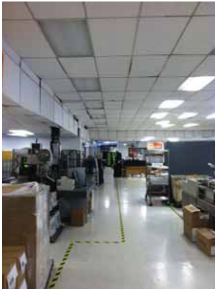
Fig. 3.0.C.2 Sagging and deteriorating 2x4 acoustic ceilings observed throughout the IDS Print Shop.
