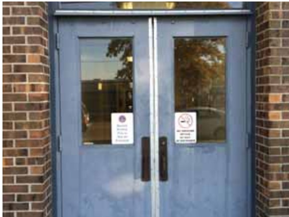
Fig. 2.1.B.18 Emergency exit equipped with a sign stating that the doors are not an entrance.
