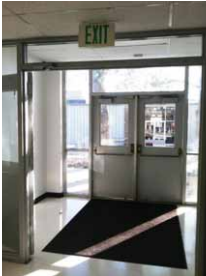
Fig. 2.1.B.4 Exit sign noted at the ceiling in front of the vestibule leading to the pair of doors on the south end of the east side of the building.
