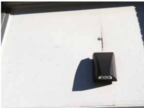
Fig. 2.1.A.20 Deteriorating paint observed at a wall panel.
