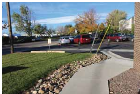
Figure 2.3.A.3 –West Entrance Walkway
