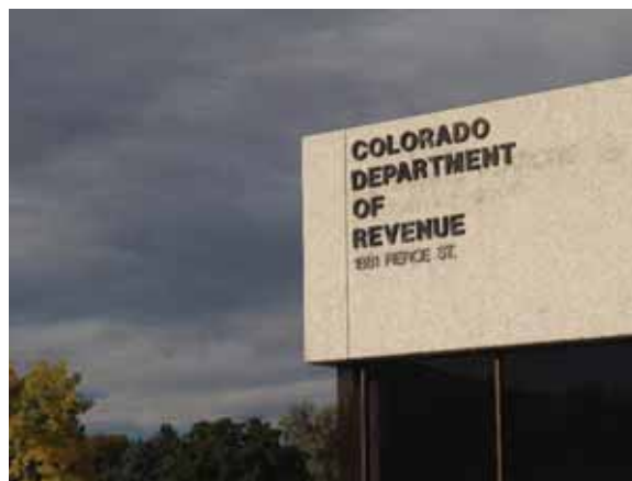
Figure 2.3.A.1 – Colorado Department of Revenue Building Exterior
