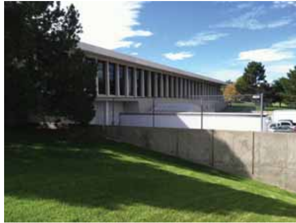
North Elevation of the 1881 Pierce Building
