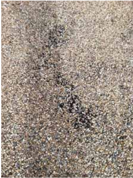
Fig. 2.1.A.44 Typical area of thin ballast.
