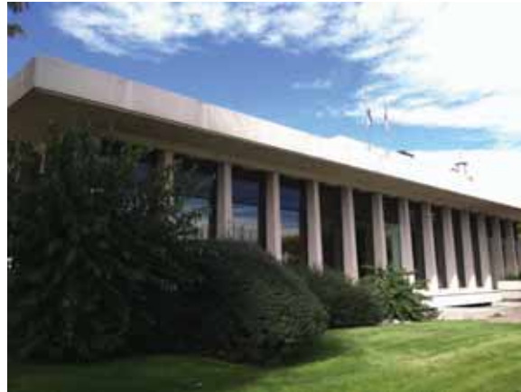
East Elevation of the north wing of the 1881 Pierce Building
