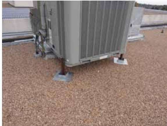
Fig. 2.4.A.25 – New Trane unit installation
