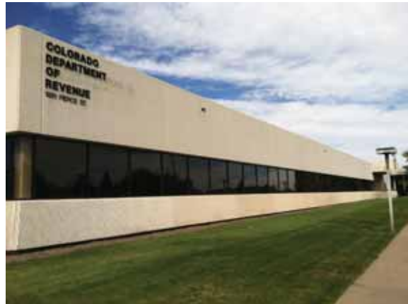
East Elevation of the south wing of the 1881 Pierce Building
