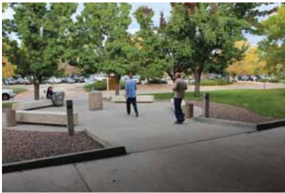
Figure 2.3.A.2 – West Entrance Concrete Walkway
