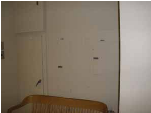
Fig. 2.4.A.3 – Panels in the wall
