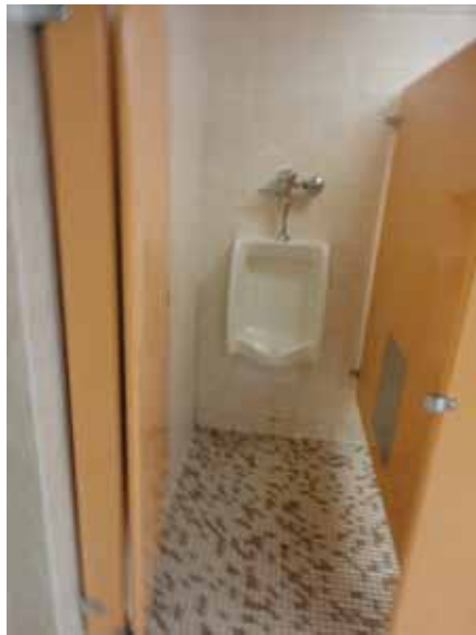
Fig. 2.1.C.2 Non-accessible urinal in the Men's First Floor Restroom located on the west side of the north wing.
