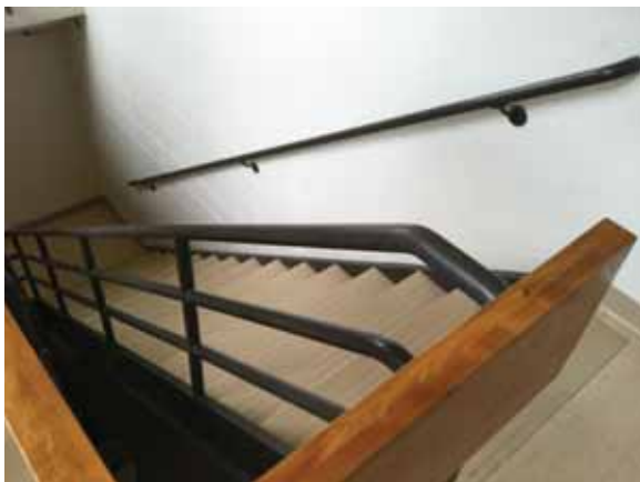
Fig. 2.1.B.5 The spacing between the guardrails in the east stairway exceeds the code-maximum of four inches.
