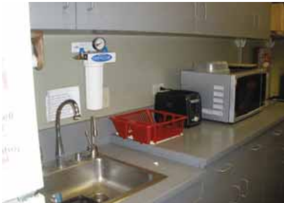
Fig. 2.4.A.15 – No GFI receptacle
