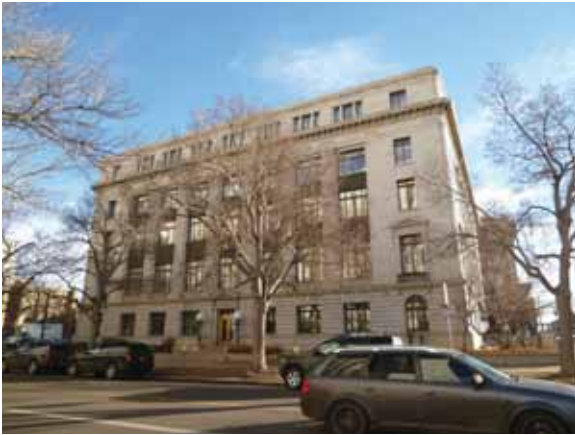
Zone 1 Exterior Facade: West elevation
