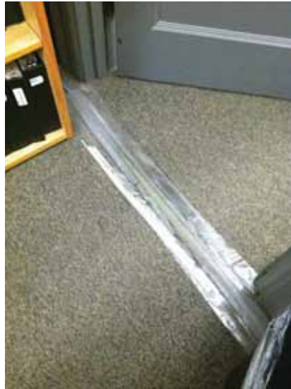
Fig. 3.1.C.34 Electrical cord taped to the floor and creating a potential tripping hazard on the Fifth Floor.
