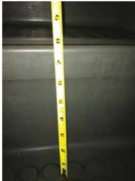
Fig. 2.1.B.6 Existing stair riser heights.
