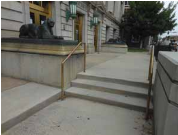
Figure 2.3.A.1 – State Office Building Colfax Avenue Entrance
