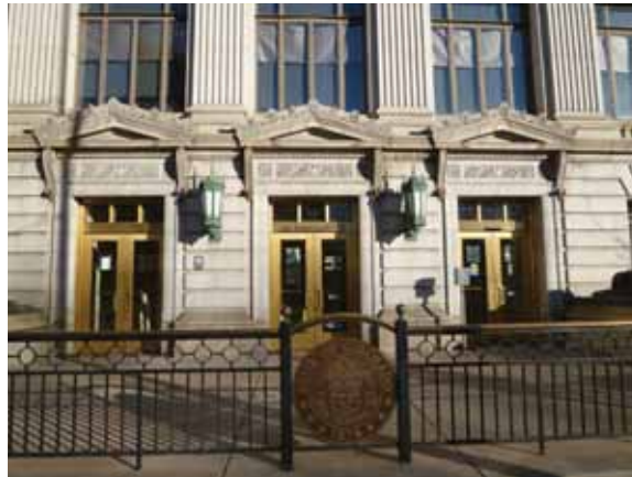
Zone 1 Exterior Facade: South entry
