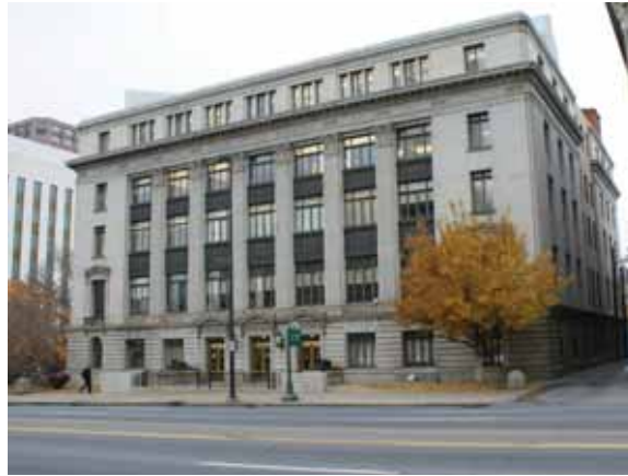
Zone 1 Exterior Facade: South and east elevations
