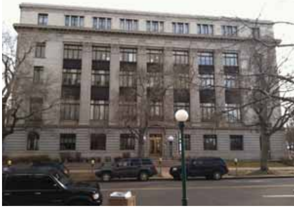
Side/West Elevation of the State Office Building
