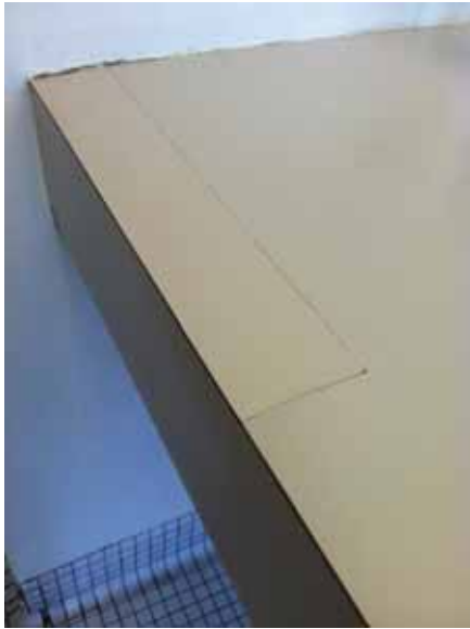
Fig. 3.1.C.42 Previously repaired section of countertop in the Women's Restroom on the Fifth Floor.
