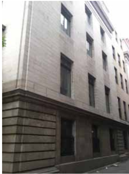
Fig. 2.1.A.6 Typical soiled granite blocks cladding the building.
