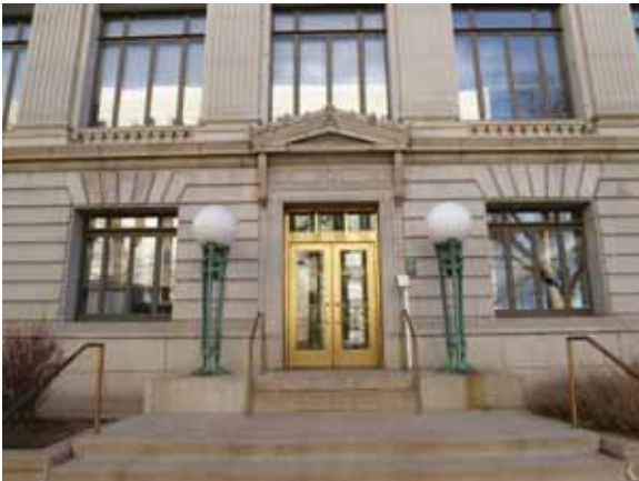
Zone 1 Exterior Facade: West entry
