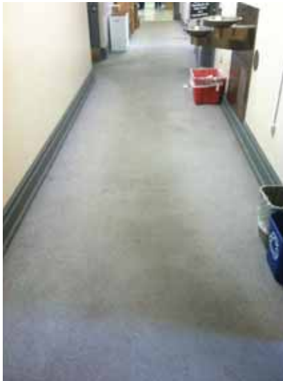
Fig. 3.1.C.32 Typical worn and soiled carpet observed in areas included in the site survey visit.
