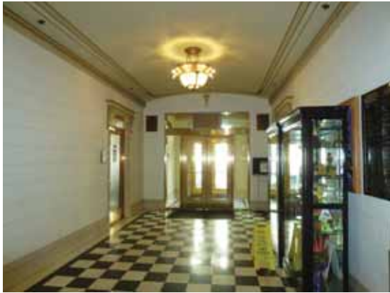
Zone 2 Interior Corridors & Circulation: Corridor connecting the west vestibule to the lobby
