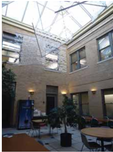
Zone 3 Central Atrium: Historic brick wall (right) and modern infill wall (left) in the atrium
