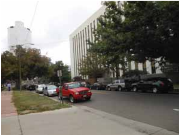
Figure 2.3.A.4 – Public Sidewalk and Treelawn on West side of Building, Looking North
