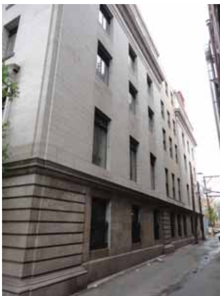
Side/East Elevation of the State Office Building
