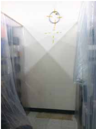
Fig. 3.1.C.25 Coiled wire taped to the wall and discolored one-foot square linoleum tile flooring in Room B-13 Library Stacks.
