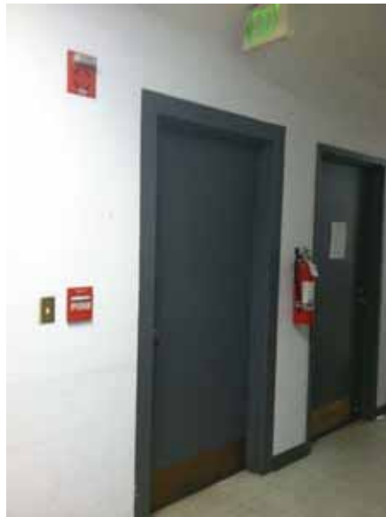
Fig. 2.1.B.4 Unmarked exit stairway door to the northeast stair from the Basement Floor.
