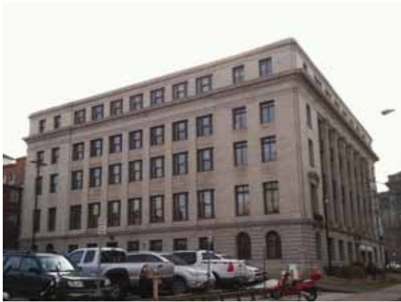
Back/North Elevation of the State Office Building
