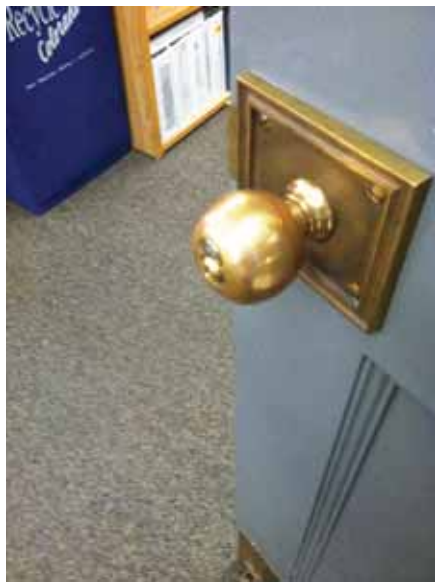
Fig. 2.1.B.12 Typical knob-style door handle found throughout the building.
