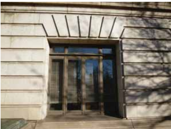
Zone 1 Exterior Facade: Typical first floor window on the south facade
