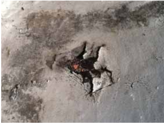
Fig. 2.1.A.22 Cracking of the painted roofing membrane.
