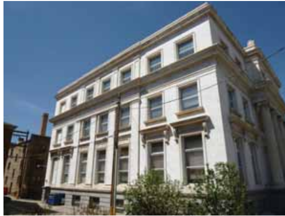
Zone 1 Exterior Facade: East elevation
