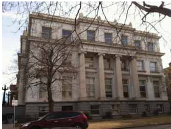
Side/West Elevation of the Legislative Services Building
