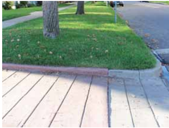
Figure 2.3.A.5 Sherman Street ROW including Sidewalk and Treelawn, looking South
