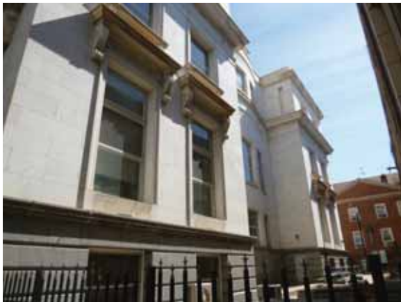
Zone 1 Exterior Facade: South elevation
