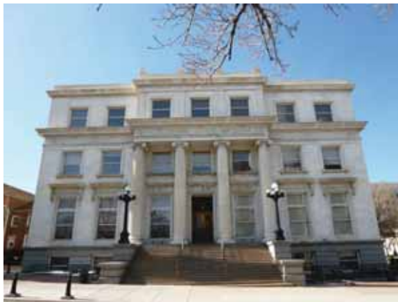
Zone 1 Exterior Facade: North elevation
