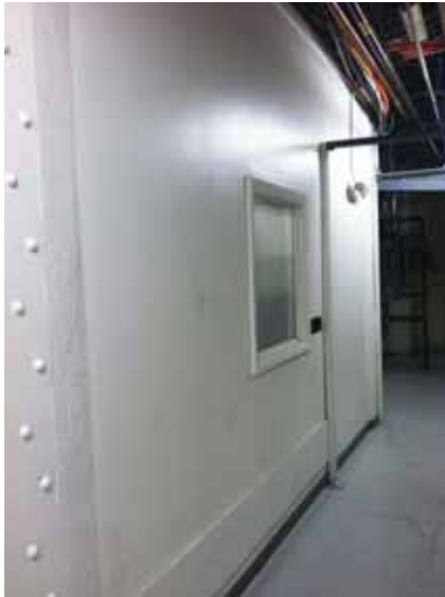
Fig. 3.1.C.14 Wear-and-tear noted to the gypsum board walls in areas of the Basement Floor included in the site survey visit.
