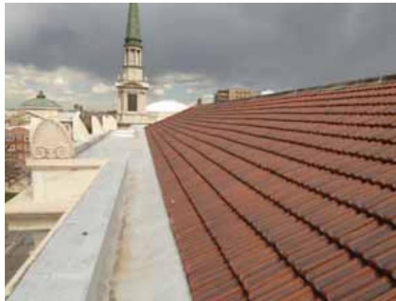
Zone 1 Exterior Facade: Red clay tile roofing
