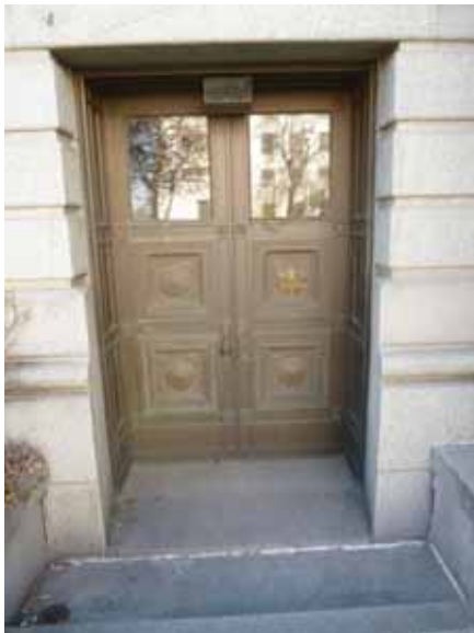
Zone 1 Exterior Facade: Ground floor entry on the west elevation
