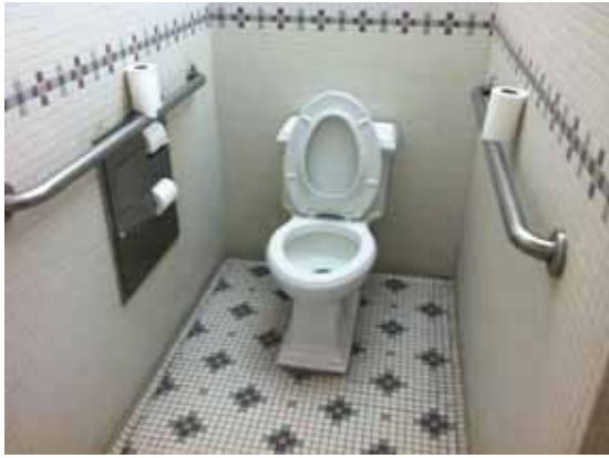
Fig. 2.1.C.1 Typical ambulatory toilet compartment.
