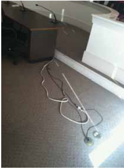
Fig. 3.1.C.24 Electrical cord creating a potential tripping hazard in the hearing room at the northeast corner of the First Floor.
