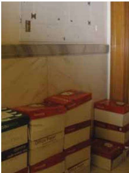
Fig. 2.4.B.4 – Boxes in front of panels
