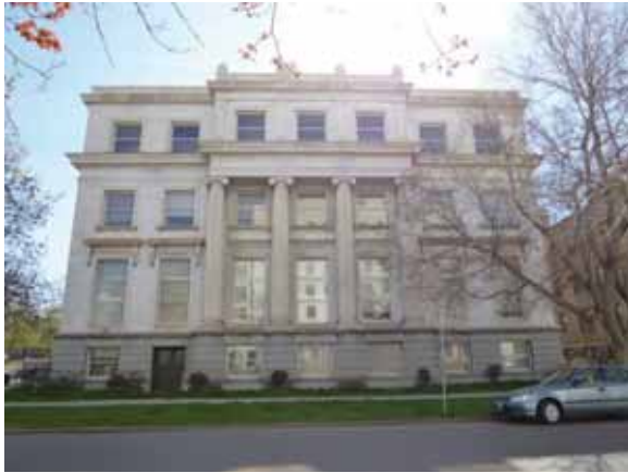
Zone 1 Exterior Facade: West elevation
