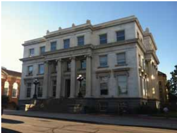
Front/North Elevation of the Legislative Services Building
