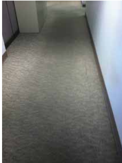
Fig. 3.0.C.17 Soiled carpet with seams pulling loose and creating a potential tripping hazard.
