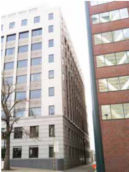
Back/West Elevation of the Human Services Building
