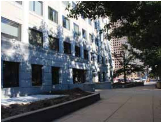
Figure 2.3.A.2 – Sherman Street Entrance Concrete Walkway
