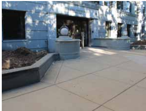
Figure 2.3.A.5 Landscape Beds at the building entrance in the process of improvement
