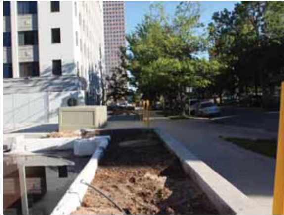
Figure 2.3.A.4 Landscape Beds in the process of improvement
