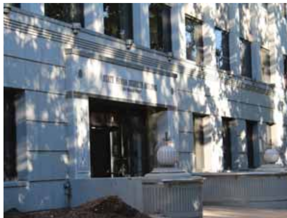
Figure 2.3.A.1 – State Human Services Building Sherman Street Entrance
