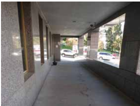
Fig. 2.1.B.8 Security camera noted at the accessible entrance on the south end of the west side of the building.
