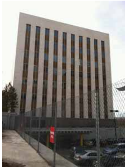
Side/North Elevation of the State Services Building
