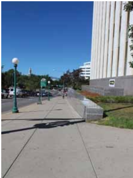
Figure 2.3.A.5 Tiered Walls along Colfax Avenue, Looking West
