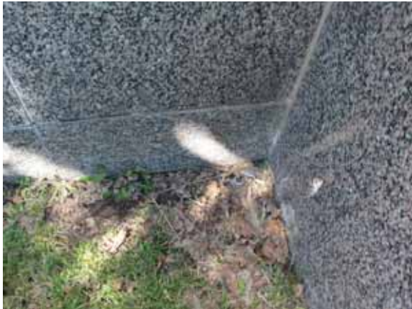
Figure 2.3.B.2 Irrigation Near Building Foundation
