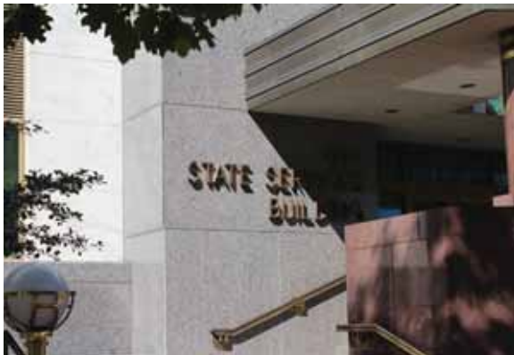
Figure 2.3.A.1 – State Services Building
