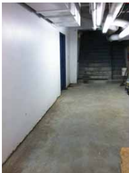
Fig. 3.0.C.22 Water damage observed at the concrete stairs and flooring near the emergency exit on the Sub-basement Floor.
