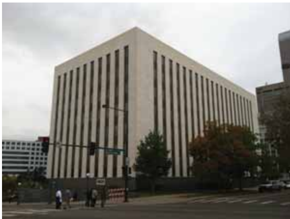
Front & Side/East & South Elevations of the State Services Building
