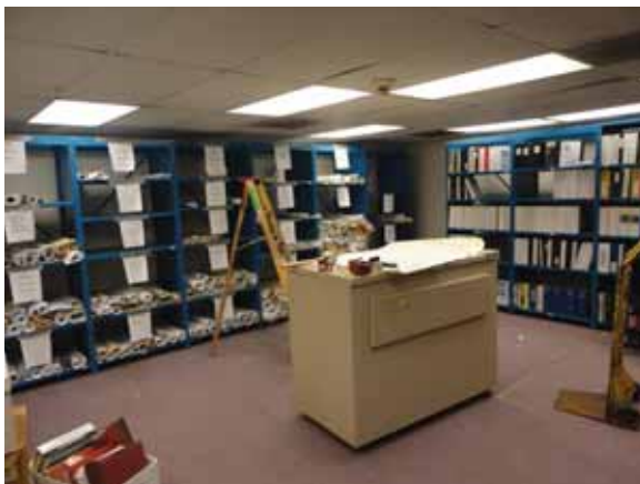
Fig. 3.0.C.14 Deteriorating and soiled carpet noted throughout the Sub-basement Floor.
