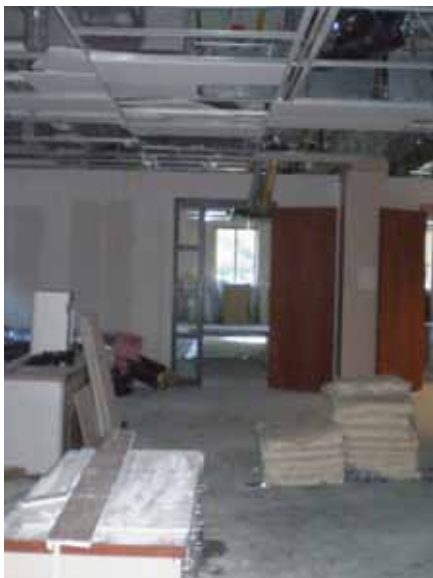
Fig. 2.4.A.1 – Remodel in progress
