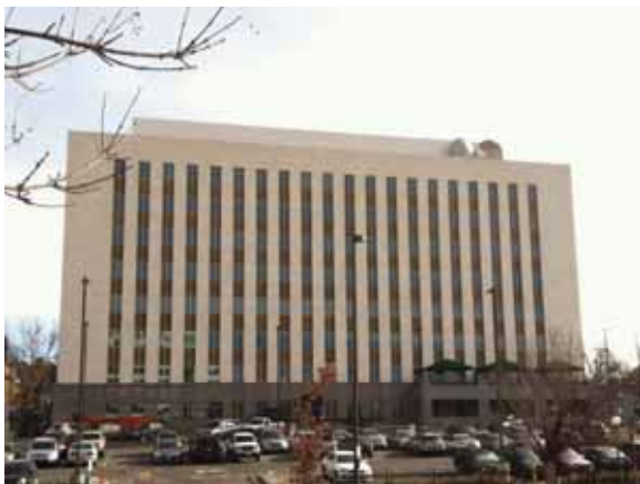
Back/West Elevation of the State Services Building
