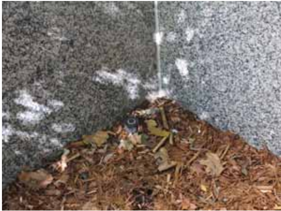
Figure 2.3.B.1 Irrigation Near Building Foundation
