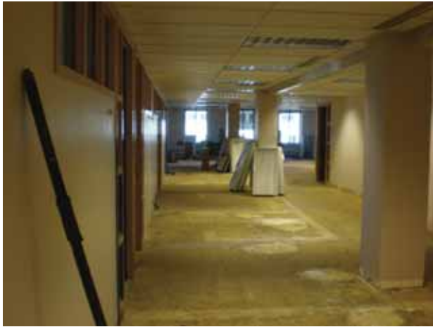
Fig. 2.4.A.5 – Light fixtures to be reused
