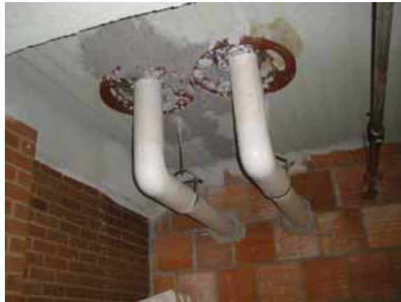
Fig. 2.4.A.13 – Roof drain piping within elevator machine room
