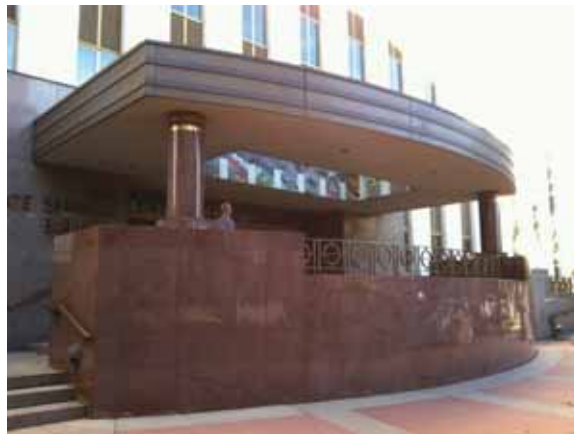
View of the Sherman Street Entrance on the east side of the building.
