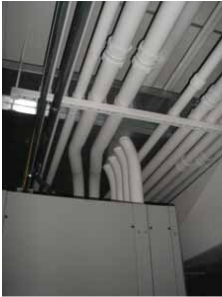
Fig. 2.4.A.21 – Drip tray over UPS
