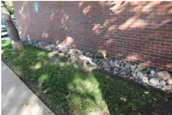
Figure 2.3.B.1– Slopes Along Building Perimeter
