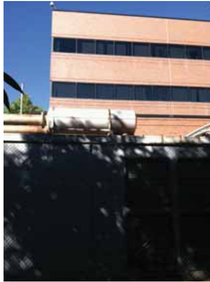
Back/East Elevation (south end) of the Dale Tooley Building
