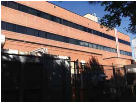
Back/East Elevation (north end) of the Dale Tooley Building
