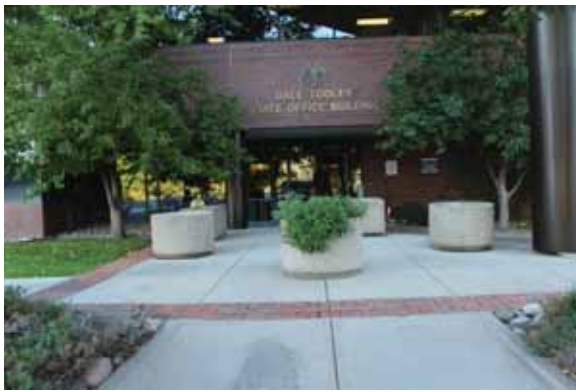
Figure 2.3.A.2 – Dale Tooley State Office Building West Entrance
