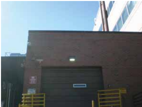
Fig 2.4.A.7 – Exterior LED light
