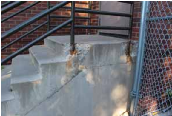
Figure 2.3.A.3 - Southeast Building Entrance
