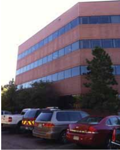
Fig. 2.1.A.2 Typical soiling of the brick observed around the perimeter of the building.
