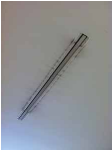
Fig. 3.0.C.1 General soiling of the gypsum board ceiling noted around the air diffusers on the First Floor.
