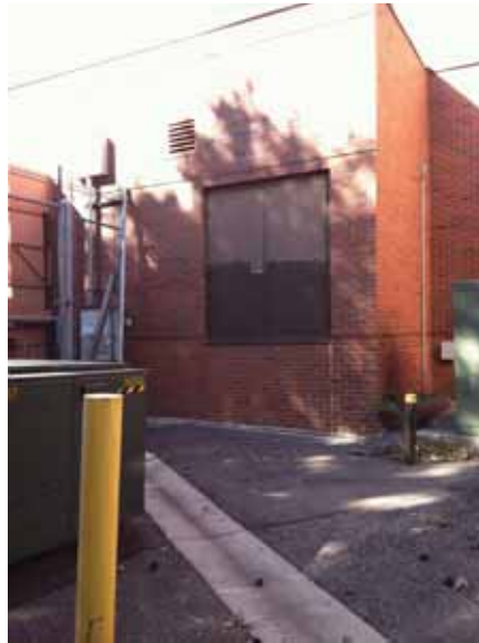
Fig. 2.1.A.8 Emergency exit doors near the middle of the east side of the building.
