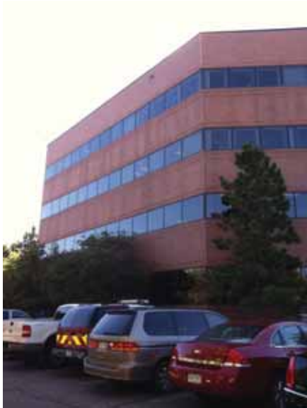
Side/North Elevation of the Dale Tooley Building
