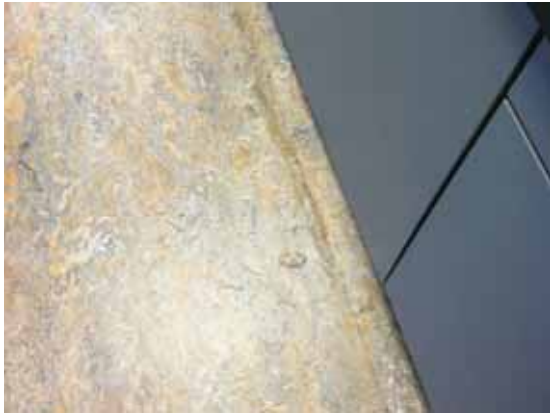
Fig. 3.0.C.30 Damage noted to the vinyl flooring in the Fourth Floor Break Room in front of the cabinets.
