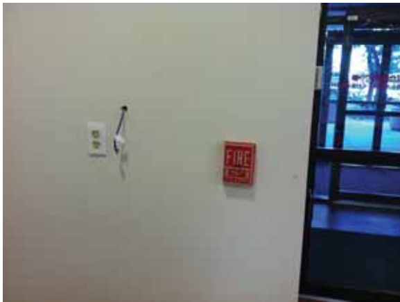
Fig. 3.0.C.10 Loose cord hanging out of a hole in the wall just to the south of the Entrance Lobby on the First Floor.
