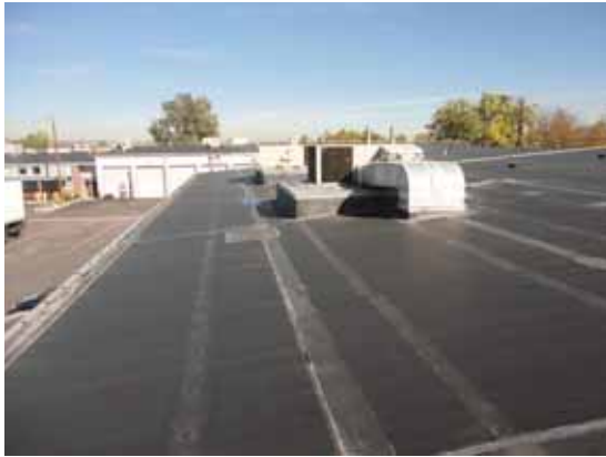
Fig. 2.1.A.14 Rubber membrane roof in fair to poor condition overall.
