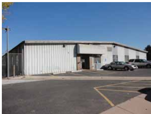
Side/South Elevation of the North Campus East Building
