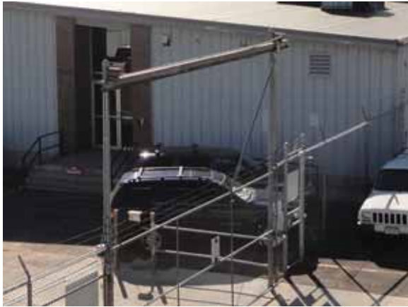
Fig. 2.1.B.15 The accessible route to and from the ramp at the entrance on the west end of the north side of the building is currently blocked by parked cars.
