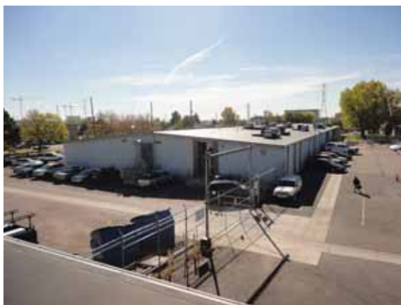
Fig. 2.1.B.16 Gated fencing controls access to the west side of the building and the majority of the North Campus site.
