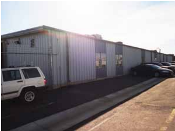
Back/West Elevation of the North Campus East Building, North End
