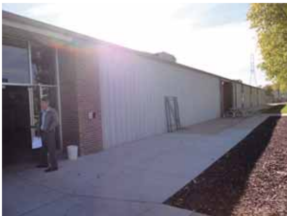
Back/West Elevation of the North Campus East Building, South End
