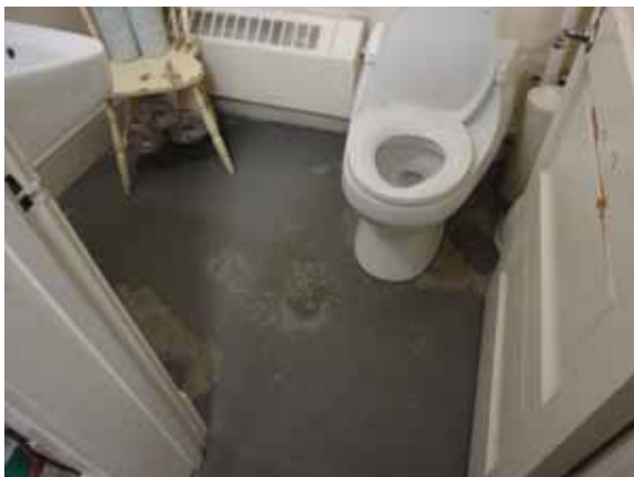
Fig. 3.0.C.34 Worn paint observed at the concrete flooring in areas throughout the Basement Floor.
