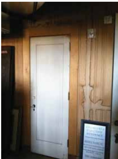
Fig. 2.1.A.35 Evidence of widespread water intrusion and damage noted throughout the attic.
