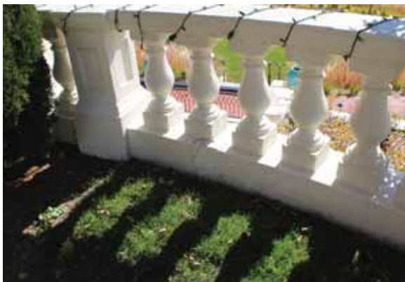
Figure 2.3.B.3 – Retaining Wall Cracking
