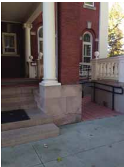
Figure 2.3.A.3 – Wheel chair accessible ramp to east entrance
