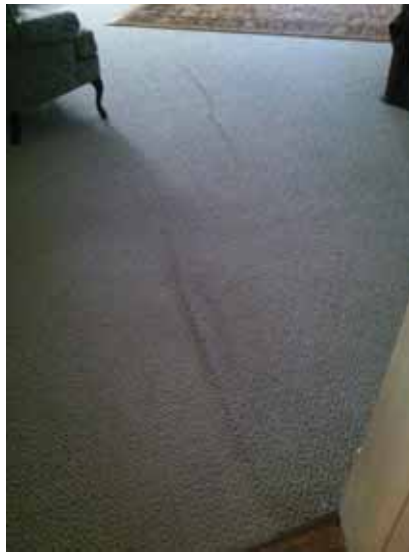
Fig. 3.0.C.24 Typical instance of carpet observed to be pulling loose and bunching, creating a potential tripping hazard, throughout the personal living quarters.
