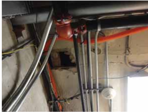
Fig. 3.0.C.5 Damage observed at areas of the plaster and wood lath ceiling on the Basement Floor.
