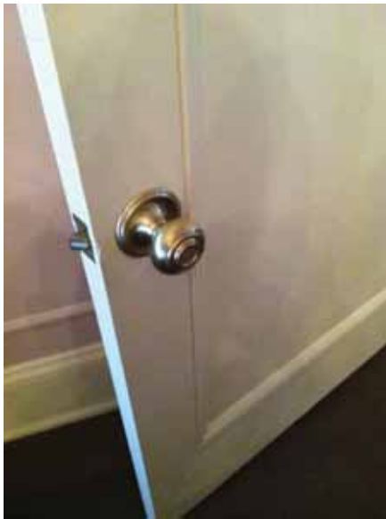
Fig. 2.1.B.6 Typical metal knob-style door handle found throughout the building.
