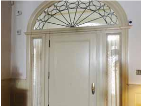
Fig. 2.1.B.8 Security alarms and detection devices observed on either side of the Front Door on the north side of the building at the First Floor.
