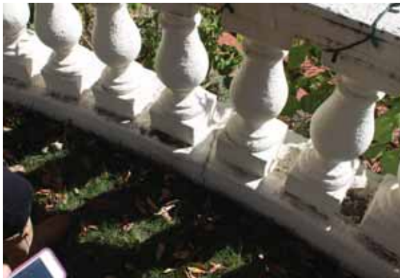
Figure 2.3.B.2 – Retaining Wall Cracking
