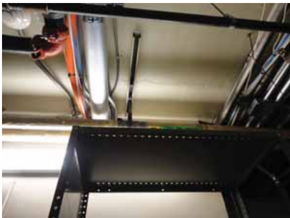
Fig. 3.0.C.4 Cracking observed at the ceiling on the Basement Floor.
