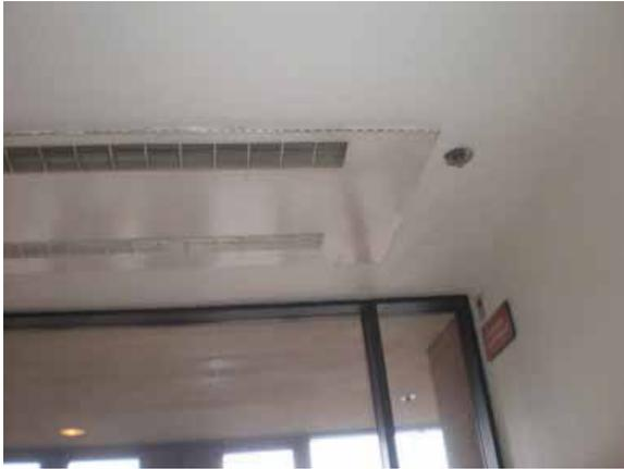
Fig. 2.4.A.33 – Sprinkler head too close to cabinet heater
