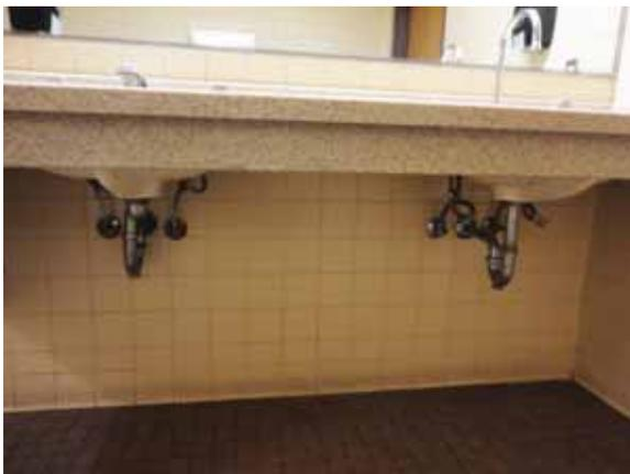
Fig. 2.1.C.5 Typical instance of an otherwise accessible lavatory without insulation wrapped around the pipes.
