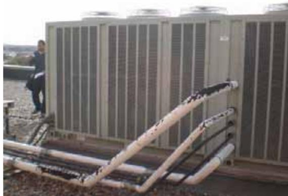
Fig. 2.4.A.13 – Trane DX condensing Unit
