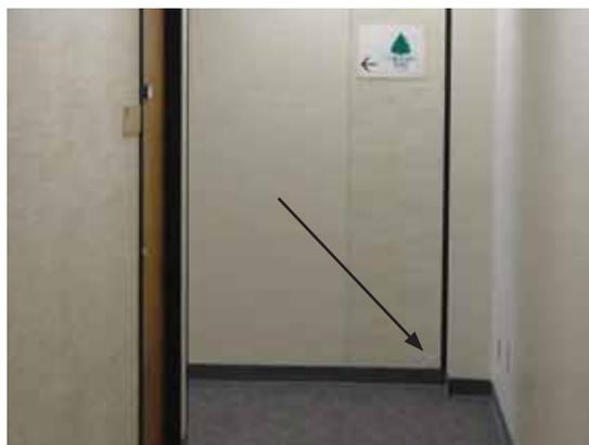
Fig. 3.0.C.5 Deteriorating and damaged wallcovering noted during the site survey visit.
