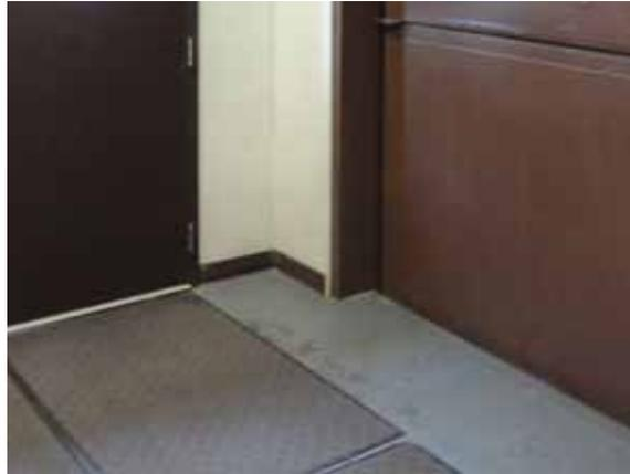
Fig. 3.0.C.13 Worn paint noted at the concrete flooring in the employee entrance and freight elevator lobby on the east end of the north side of the First Floor.
