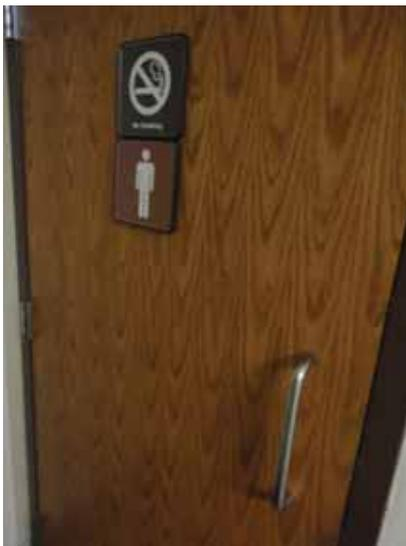
Fig. 2.1.B.7 Typical pull-style door handle noted at the restroom doors.
