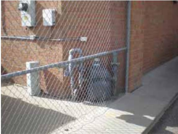
Fig. 2.4.A.34 – Electrical meter close to gas meter
