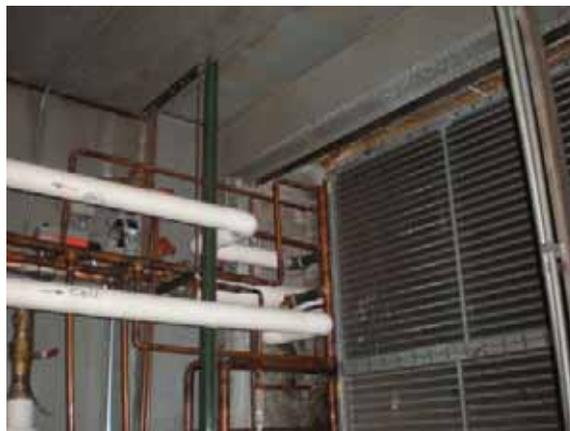
Fig. 2.4.A.20 – Built-up AHU hot water heating coil
