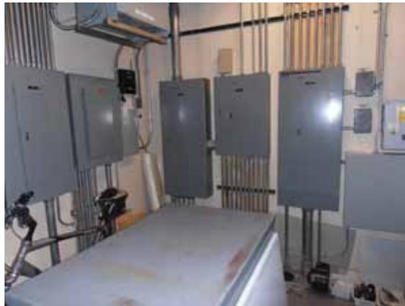
Fig. 2.4.A.3 – Panels and transformers
