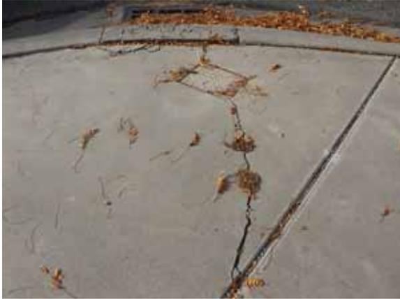
Figure 2.3.A.4 – Site Concrete Crack, Recommended for Replacement
