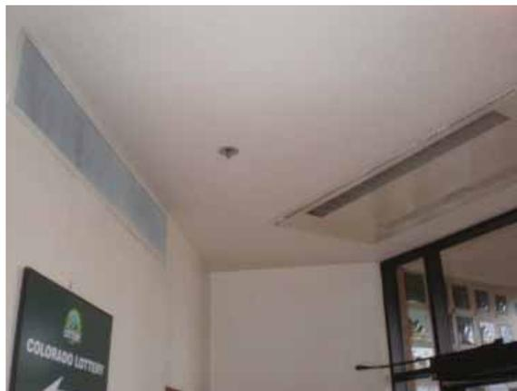
Fig. 2.4.A.32 – Sprinkler head close to cabinet heater
