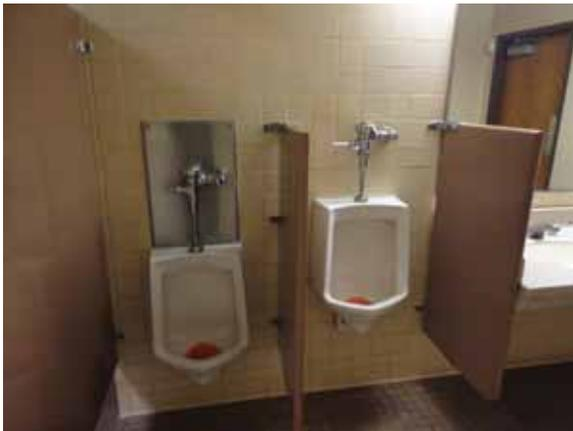
Fig. 2.1.C.4 The width of the urinal alcove is too narrow per accessibility standards.
