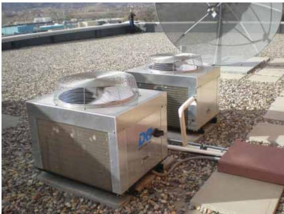
Fig. 2.4.A.16 – Data Air condensing units
