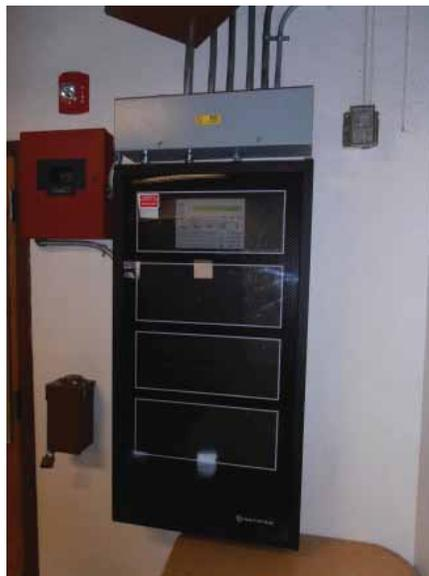
Fig. 2.4.A.8 – Fire alarm control panel
