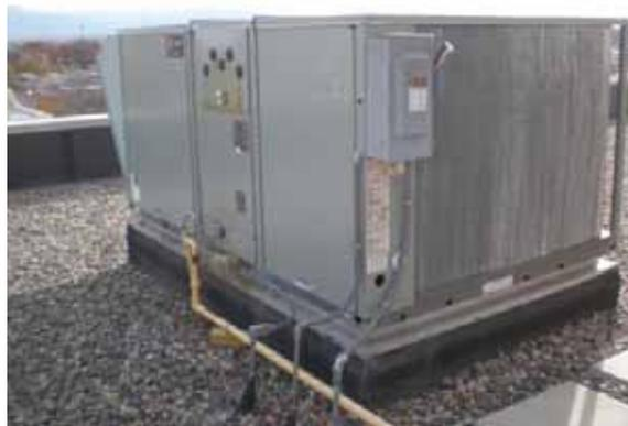
Fig. 2.4.A.14 – Trane RTU serving microwave server room
