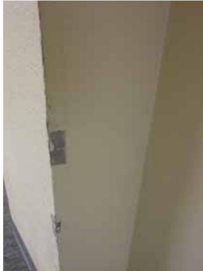
Fig. 3.0.C.3 General wear-and-tear at areas of the gypsum board walls noted on the Third Floor.
