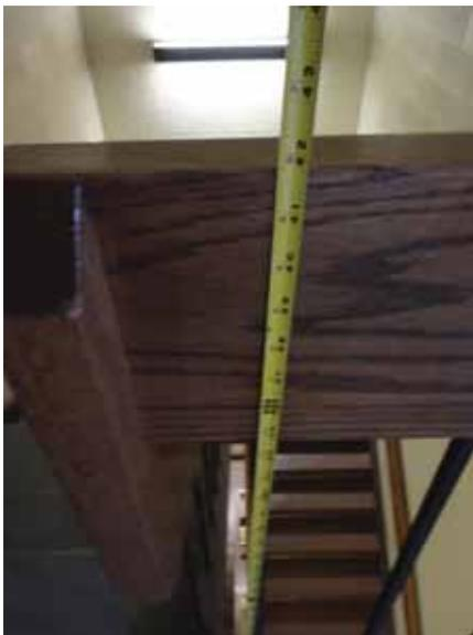
Fig. 2.1.B.3 The height to the top of the guardrail within the interior exit stairways.
