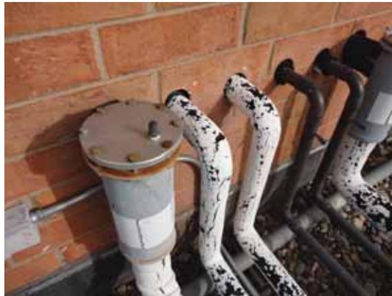
Fig. 2.1.A.5 Unsealed openings around pipe penetrations at a portion of the brick walls at the Penthouse are exposing the building envelope to water penetration.
