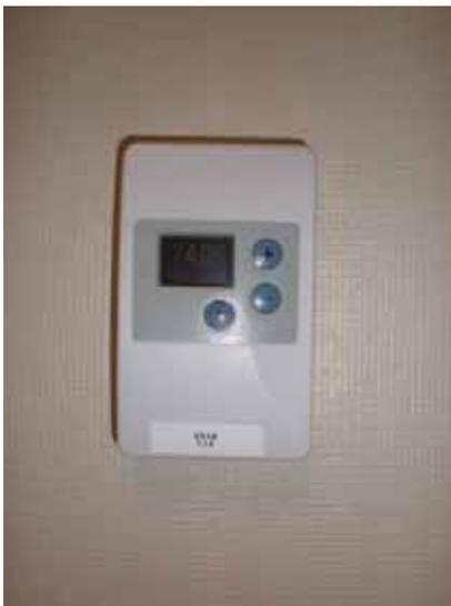
Fig. 2.4.A.23 – Digital space temperature sensor
