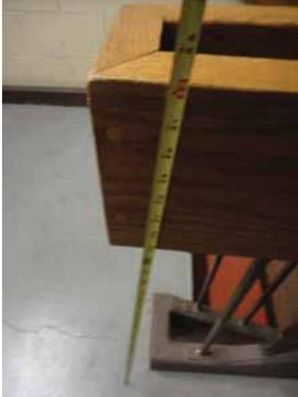
Fig. 2.1.B.2 The height to the top of the handrail measured above the stair tread nosing.
