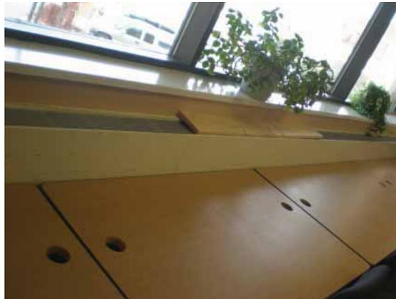
Fig. 2.4.A.31 – Baseboard outlet blocked with wood
