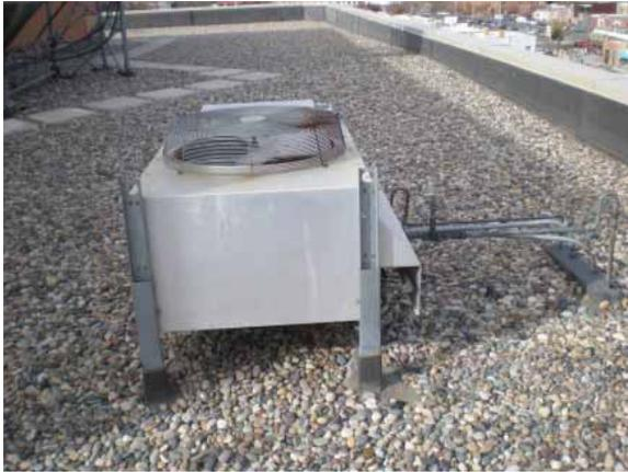
Fig. 2.4.A.15 – Condensing unit serving telecom room
