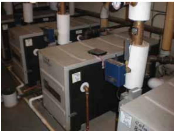
Fig. 2.4.A.17 – Hot Water Boilers
