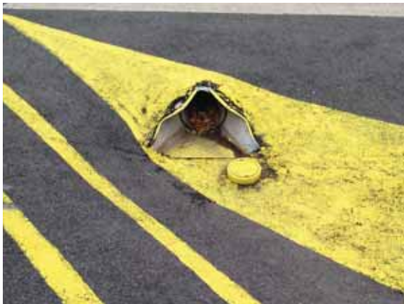
Figure 2.1.A.18 – Small Culvert in Roadway
