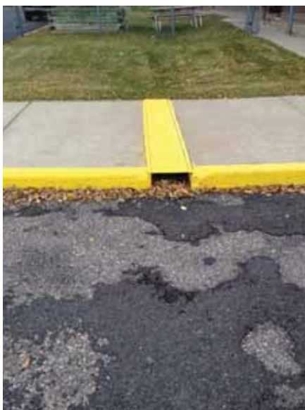
Figure 2.1.A.12 – Curb Cut through Sidewalk near Building #120
