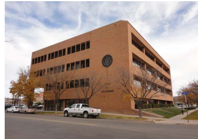
Grand Junction State Services Building
