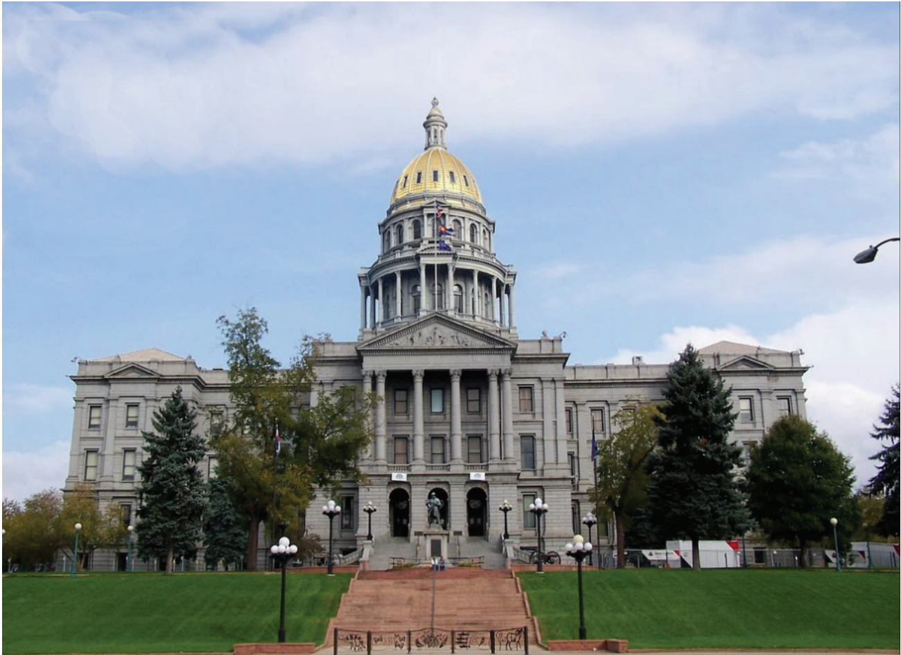
Illustration D: Showing the Capitol building and West Lawn From Lincoln Street with Schuetze's Central Walkway in the Foreground
