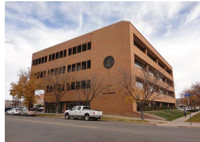
Grand Junction State Services Building
