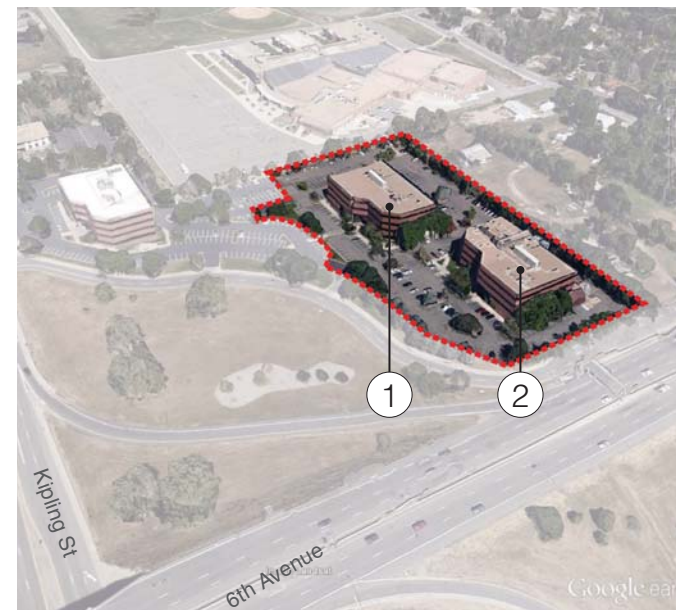
Oblique View of the Kipling Campus
