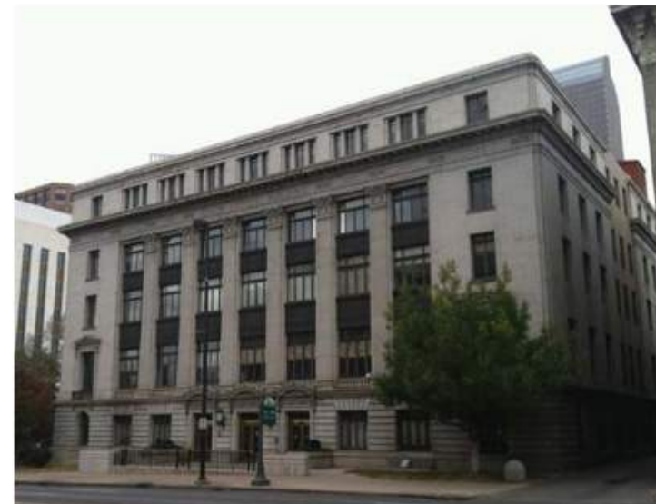
201 E. Colfax St., State Office Building
