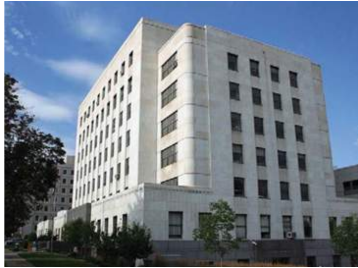
Annex Building (Currently Vacant)
