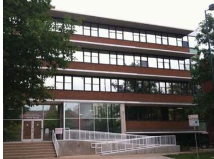
1570 Grant Building (Currently Vacant)
